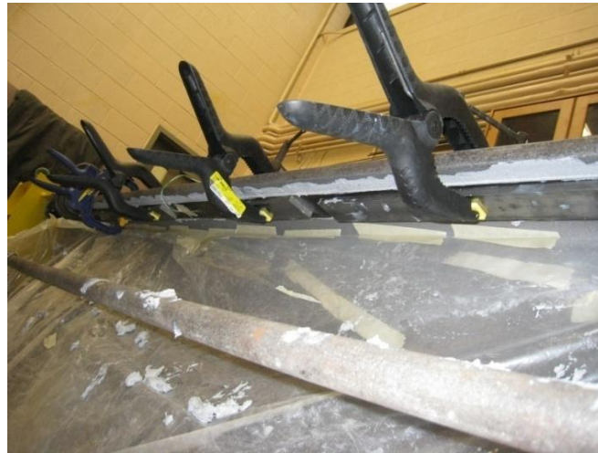
Figure 3.13. CFRP strip clamped to the beam after prestressing
