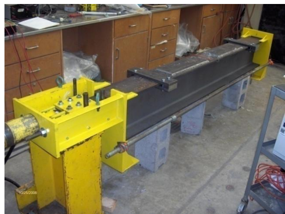
(b) Completed prestressing system for the strips on the inner side of the flange.
