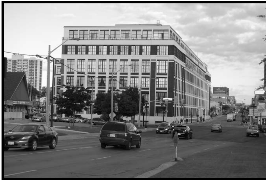
Kaufman Lofts (King St S), Constructed: 2007. Kitchener waived $1.4 Million development charges fee Photo by Adam Lauder
