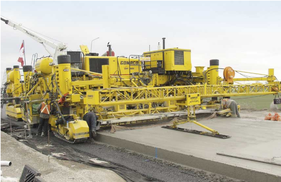
Figure 2.3: Dowel Bar Inserter in action on Highway 401, Ontario, Canada [16]
