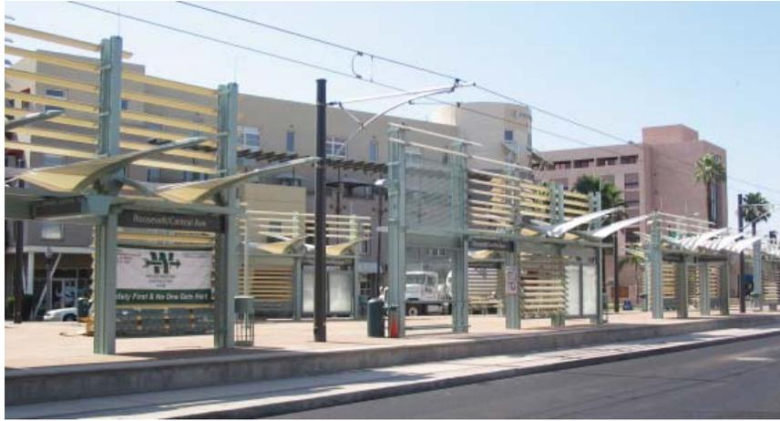
The station design responds to Arizona's desert climate. Louvered panels and overhead canopies are used to maximize shade and comfort at all times of day. Cool-surface paint is used to protect furniture from overheating. Collaborating with local artists, unique public art pieces are integrated with selected stations.
