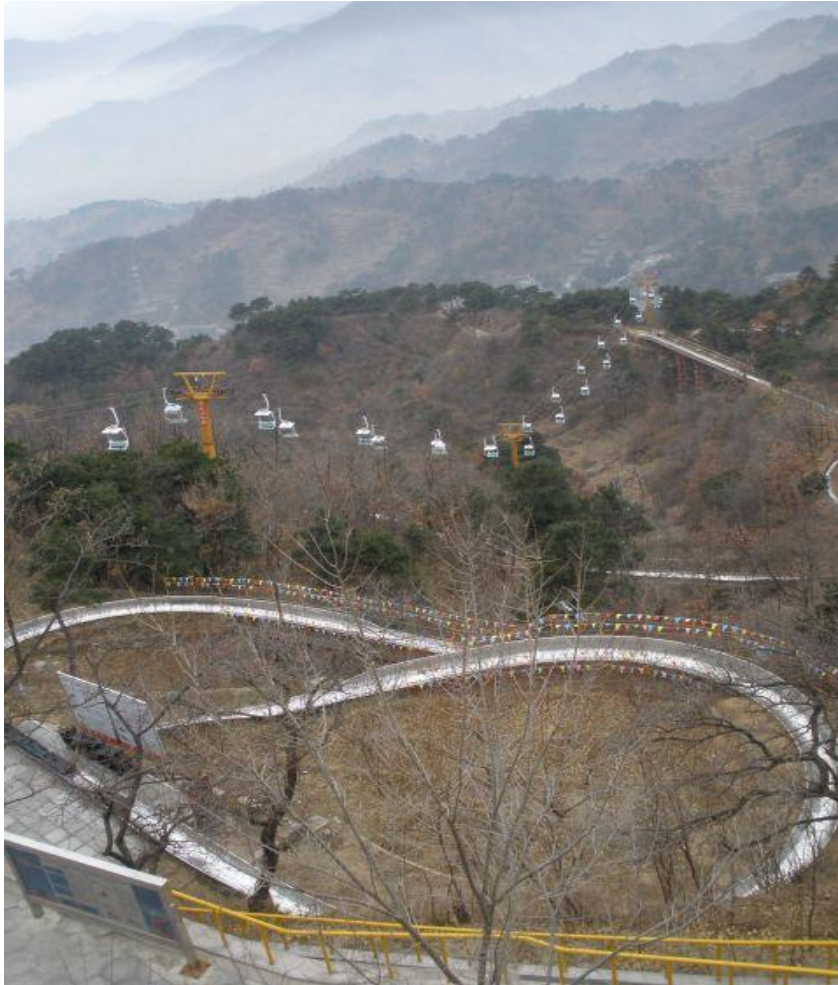
Figure 6.6: Overview of the cable car and slide way on top of the Mutianyu Great Wall
