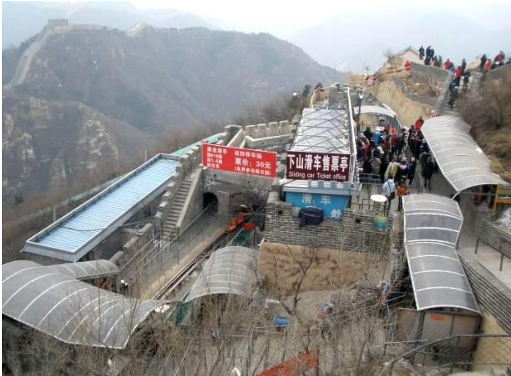
Figure 5.29: Slideway station at North Watchtower Five
