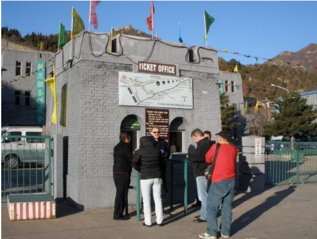
Figure 5.25: Cable Car ticket office at Guntiangou parking lot
