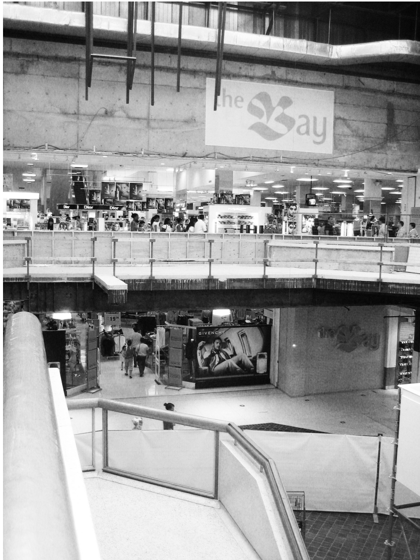
fig 4.15 (above) Scarborough Town Centre, under construction, summer 2009.
