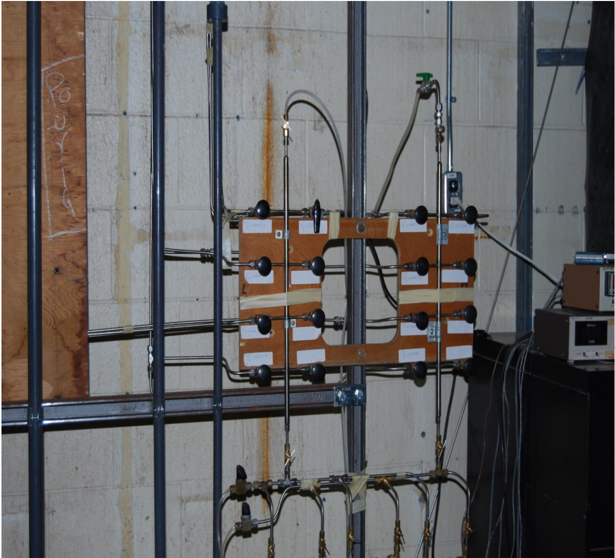
Figure 4.4 View of pressure transducers manifolds and tubing
