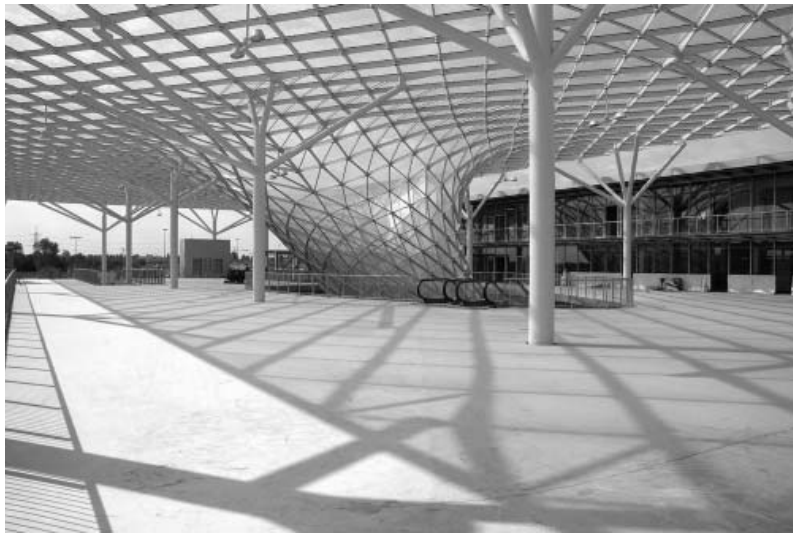
fig. 76. In the Fiera di Milano Exhibition Centre, Massimiliano Fuksas distributed public amenities and attractions along a raised central walkway seven metres above ground to differentiate them from the private exhibitions below.
