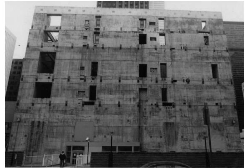
fig. 12. The core’s north elevation.
