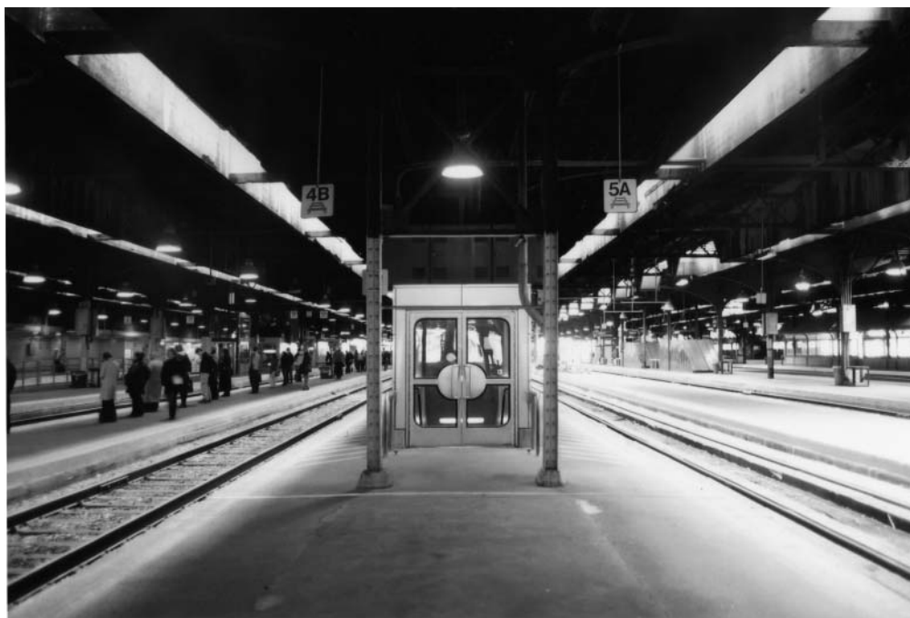
fig. 33. Stair vestibule on Platform 4B and 5A
