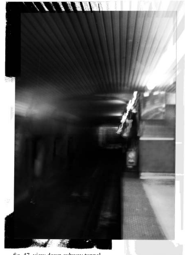
fig. 47. view down subway tunnel
