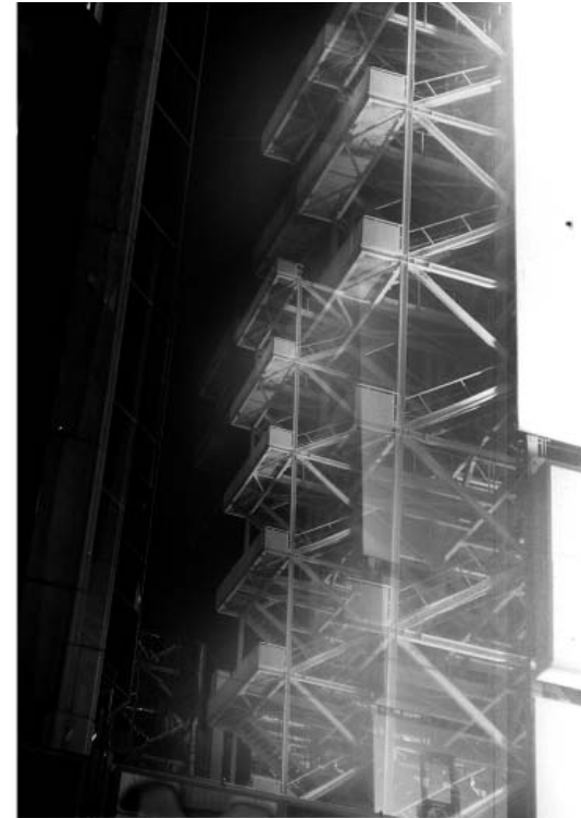
fig. 59. media tower stairs
