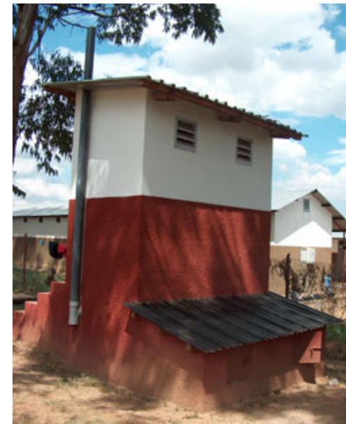
Figure 6.19 A composting pit latrine is vented, and raised above the ground to provide access to the vaults below. The metal sheet heats up and aids decomposition
