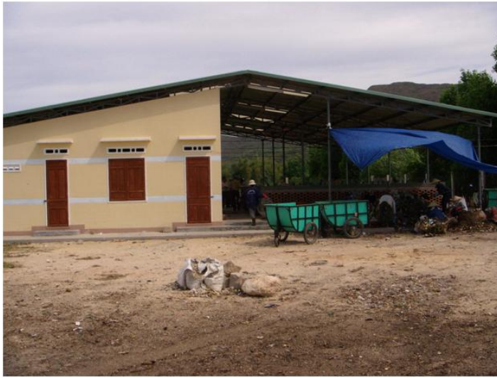
Photo 7 - Quy Nhon small-scale composting plant
