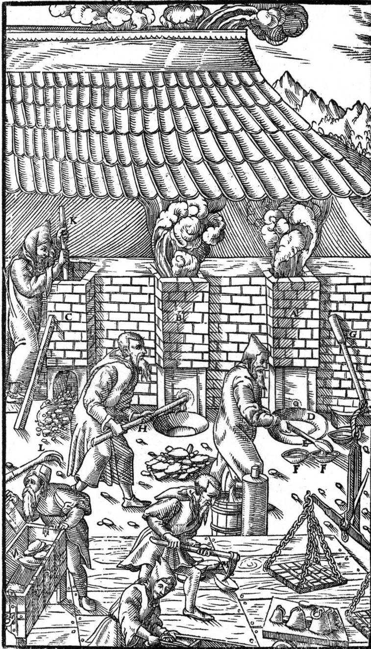
Fig. 54. Three smelting furnaces in operation. At A, right, the smelter pours the molten metal from the forehearth into iron or copper molds. The man behind him opens the tap-hole of the middle furnace with a tapping-bar. The third man is cleaning furnace C. In the foreground are a strong chest and weighing scales.
