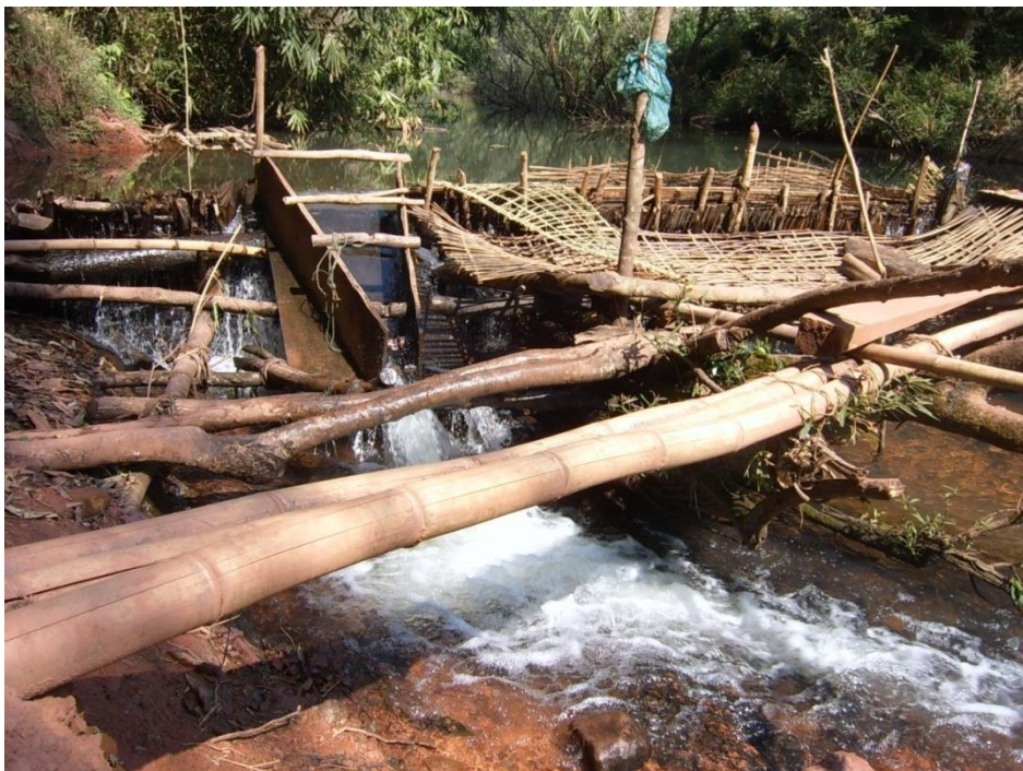
PHOTO 1: EXAMPLE OF MULTIPURPOSE DAM FROM VILLAGE B FOR HYDRO-ELECTRICITY GENERATION, WATER DETENTION AND CATCHING FISH.
