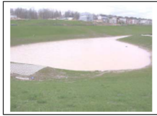
Picture of a newly constructed Storm Water Management Pond
