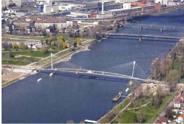
Figure 11 View on pedestrian bridge in Two Shores Garden ( www.france-for-visitors.com )
