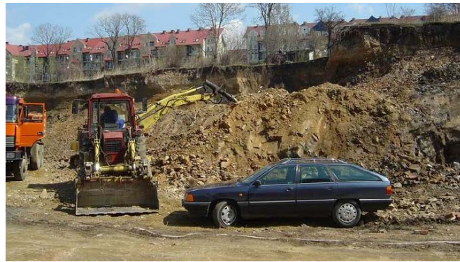
Figure 32 Implementation of project of Zgorzelec Postal Market rebuilding
