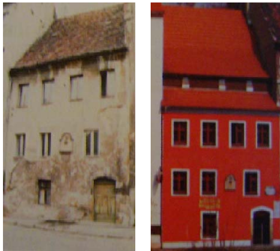
Figure 25 Photographs of the Böhme House made before (on left) and after (on right) renovation (Europamiasto Görlitz-Zgorzelec, 2006, p.5)
