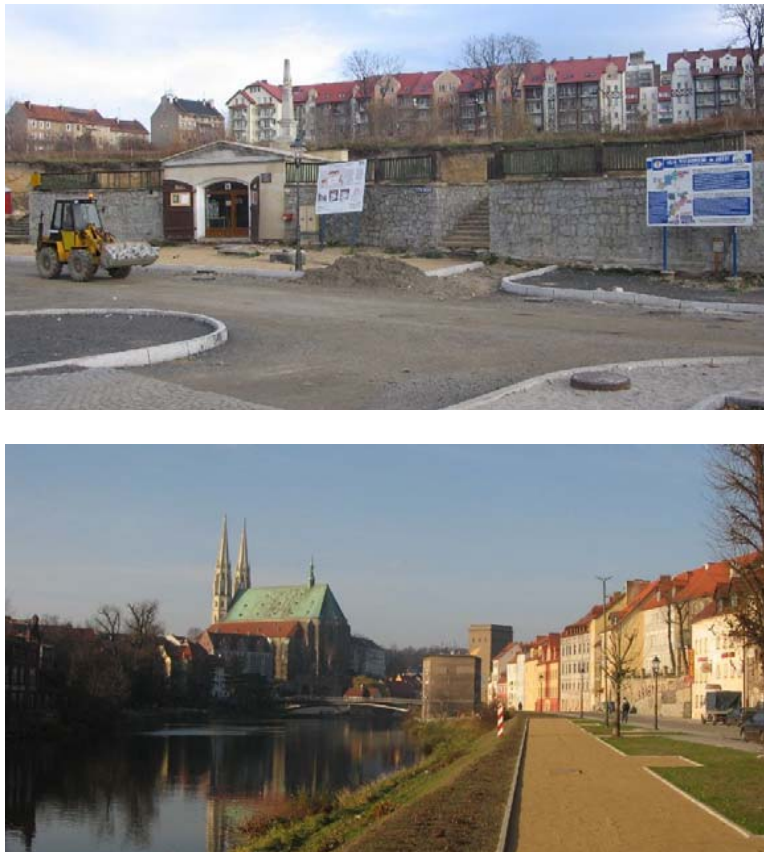
Figure 33 Restoration of roads and sidewalks in Zgorzelec Old Town (personal sources)
