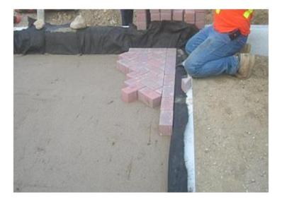
**Figure 19: ICP Placement**
