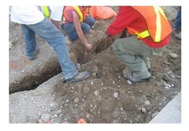
**Figure 41: Temperature Probe Installation**
