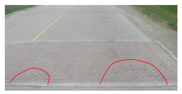
Figure 79: Depressions, Ruttings and Joint Sand Loss and in SSCBCH
