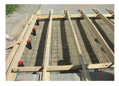
Figure 16: Formworks, Drain Pipes and Reinforcement Bars for BSCBCH
