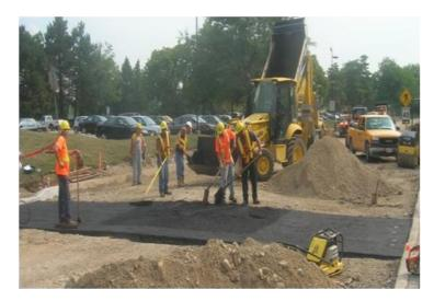
Figure 33: Asphalt Base Construction
