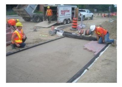
**Figure 35: Interlocking Concrete Pavers Placement**
