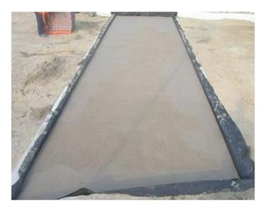
Figure 17: Bedding Sand and Non-Woven Geotextile
