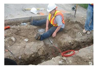
Figure 40: Earth Pressure Cells Installation
