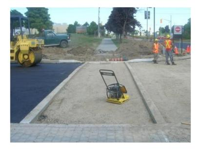
Figure 34: Granular Base Construction
