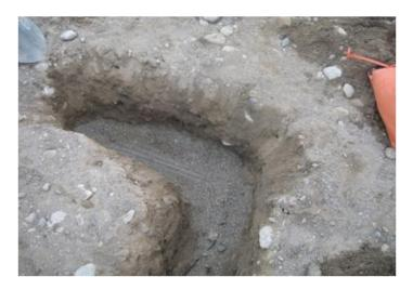
**Figure 39: Moisture Probes Installation**
