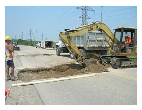
Figure 12: Excavation of Existing Asphalt Pavement
