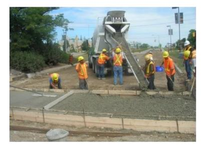
**Figure 31: Concrete Placement on SSCBCH Section**
