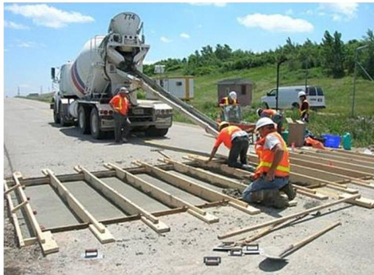
**Figure 13: Concrete Placement on BSCBCH**
