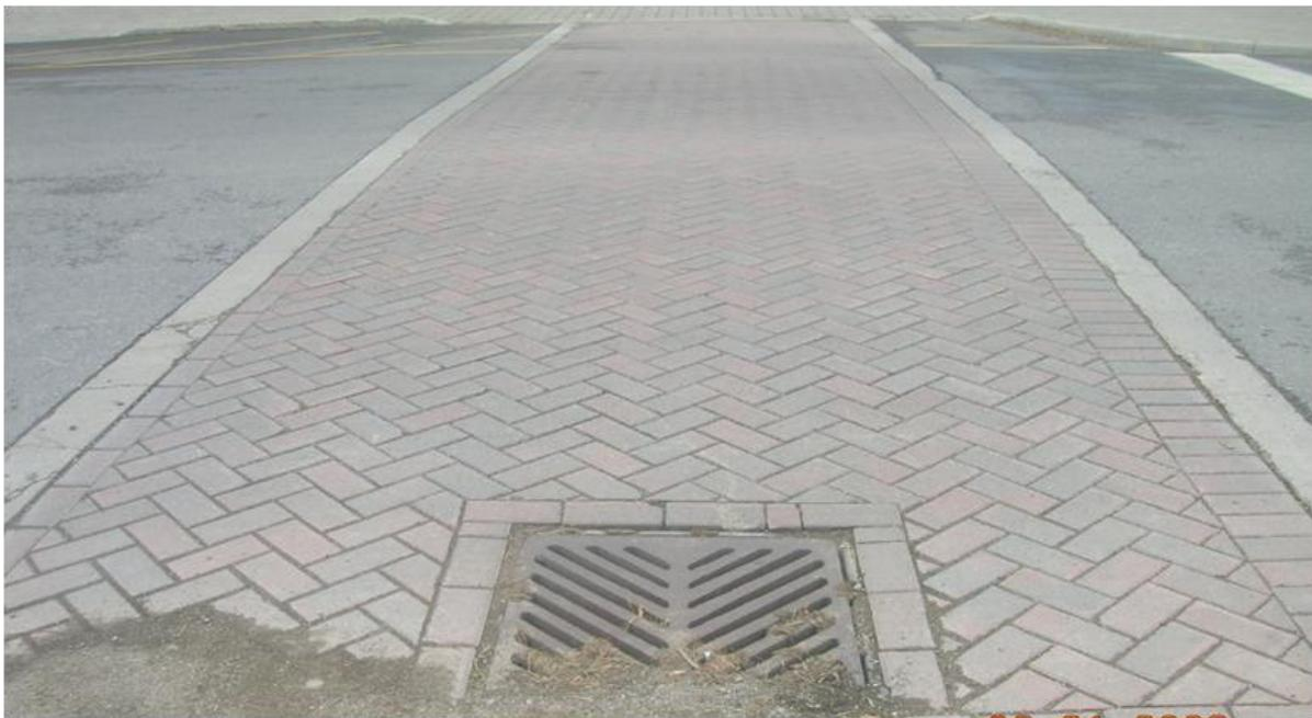
**Figure 97: Uniform Deformations and Cracks on Concrete Headers in SGBCH**
