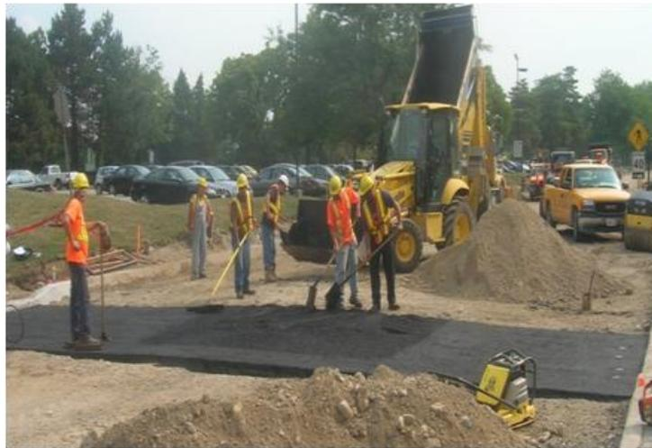
**Figure 33: Asphalt Base Construction**
