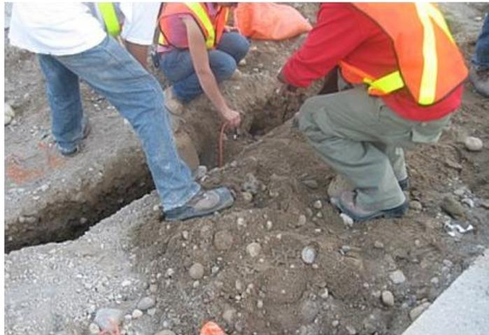
**Figure 41: Temperature Probe Installation**
