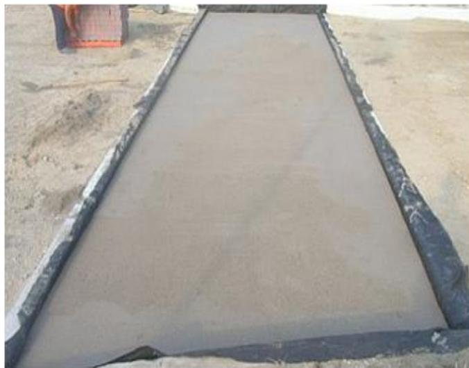
**Figure 17: Bedding Sand and Non-Woven Geotextile**
