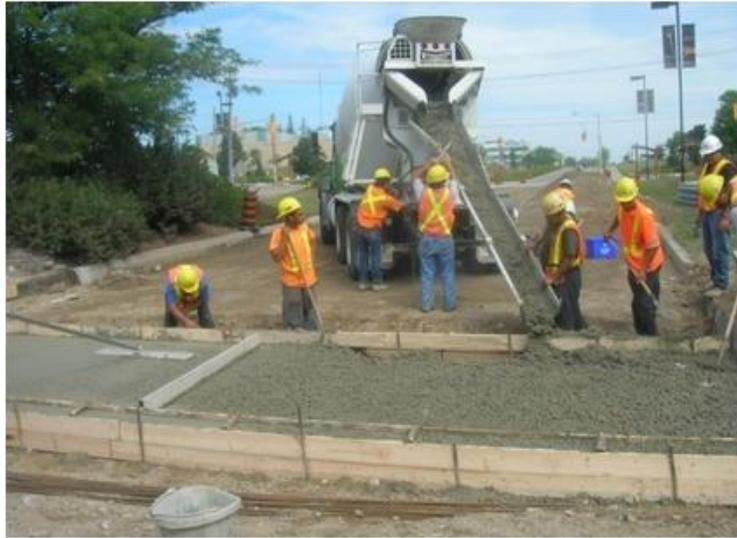
**Figure 31: Concrete Placement on SSCBCH Section**
