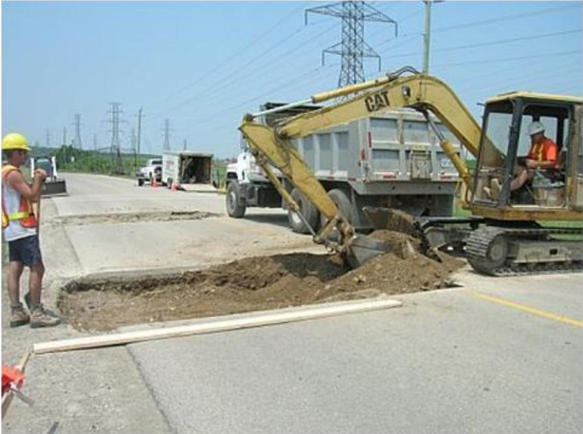
**Figure 12: Excavation of Existing Asphalt Pavement**
