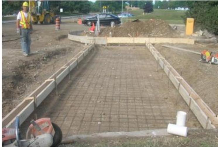
**Figure 30: Formworks, Drainage Pipes and Reinforcement Bars for SSCBCH Section**
