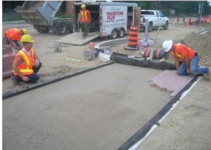
**Figure 35: Interlocking Concrete Pavers Placement**
