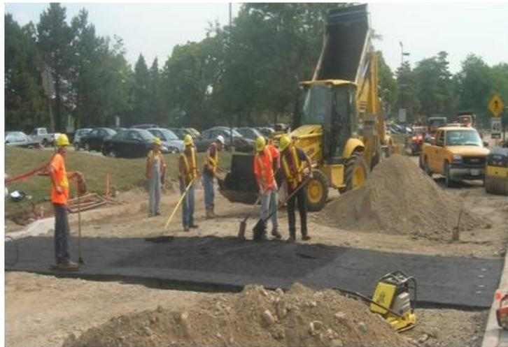
**Figure 33: Asphalt Base Construction**
