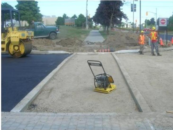
**Figure 34: Granular Base Construction**
