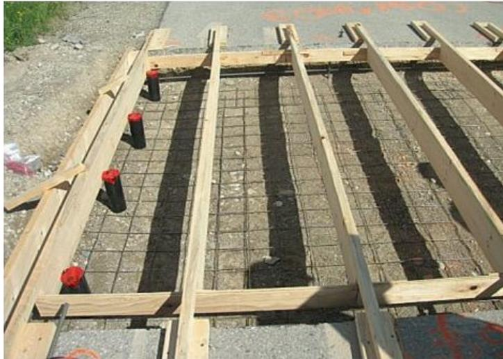
**Figure 16: Formworks, Drain Pipes and Reinforcement Bars for BSCBCH**
