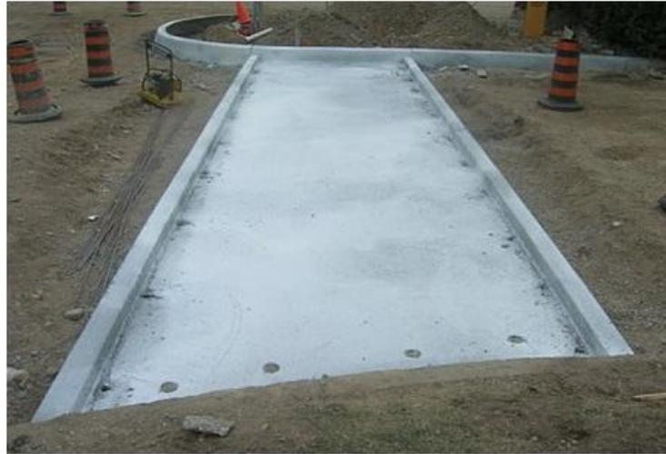
**Figure 32: Concrete Base Section**
