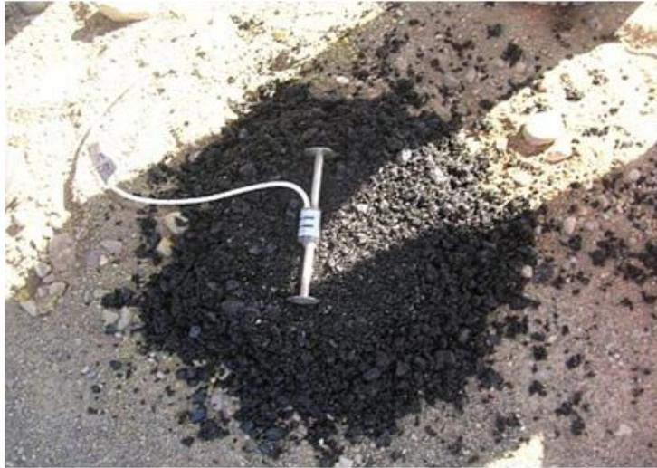
**Figure 44: Vibrating Wire Asphalt Strain Gauge Installation**
