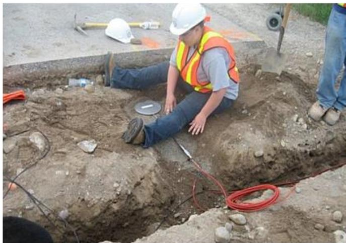
**Figure 40: Earth Pressure Cells Installation**
