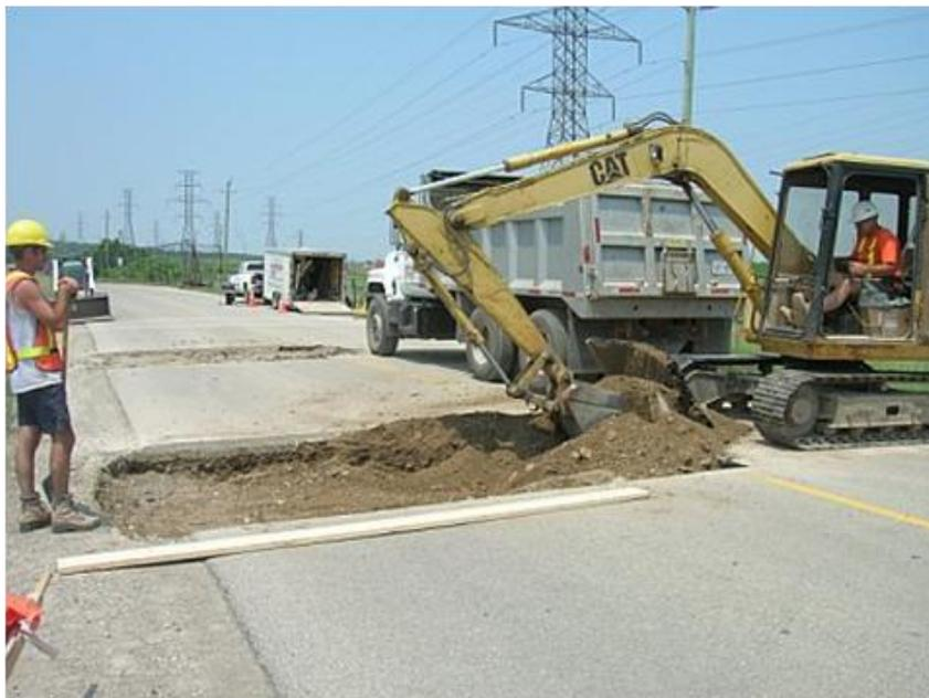
**Figure 12: Excavation of Existing Asphalt Pavement**
