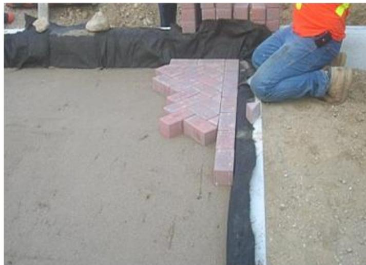
**Figure 19: ICP Placement**
