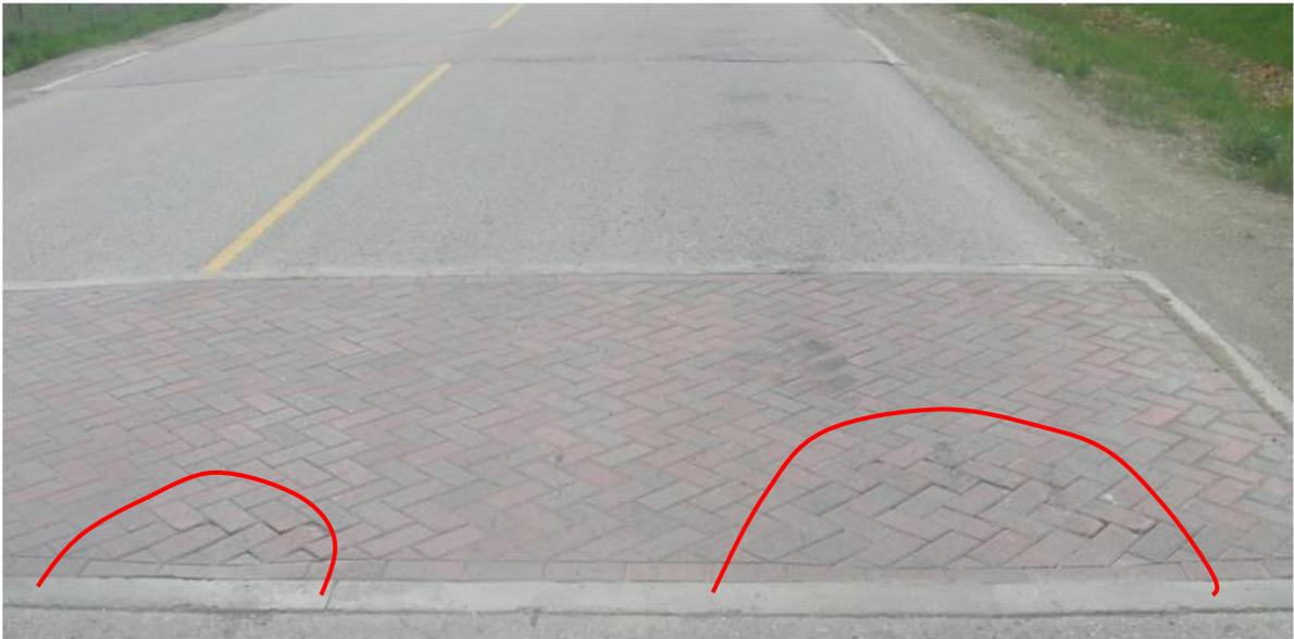
**Figure 79: Depressions, Ruttings and Joint Sand Loss and in SSCBCH**
