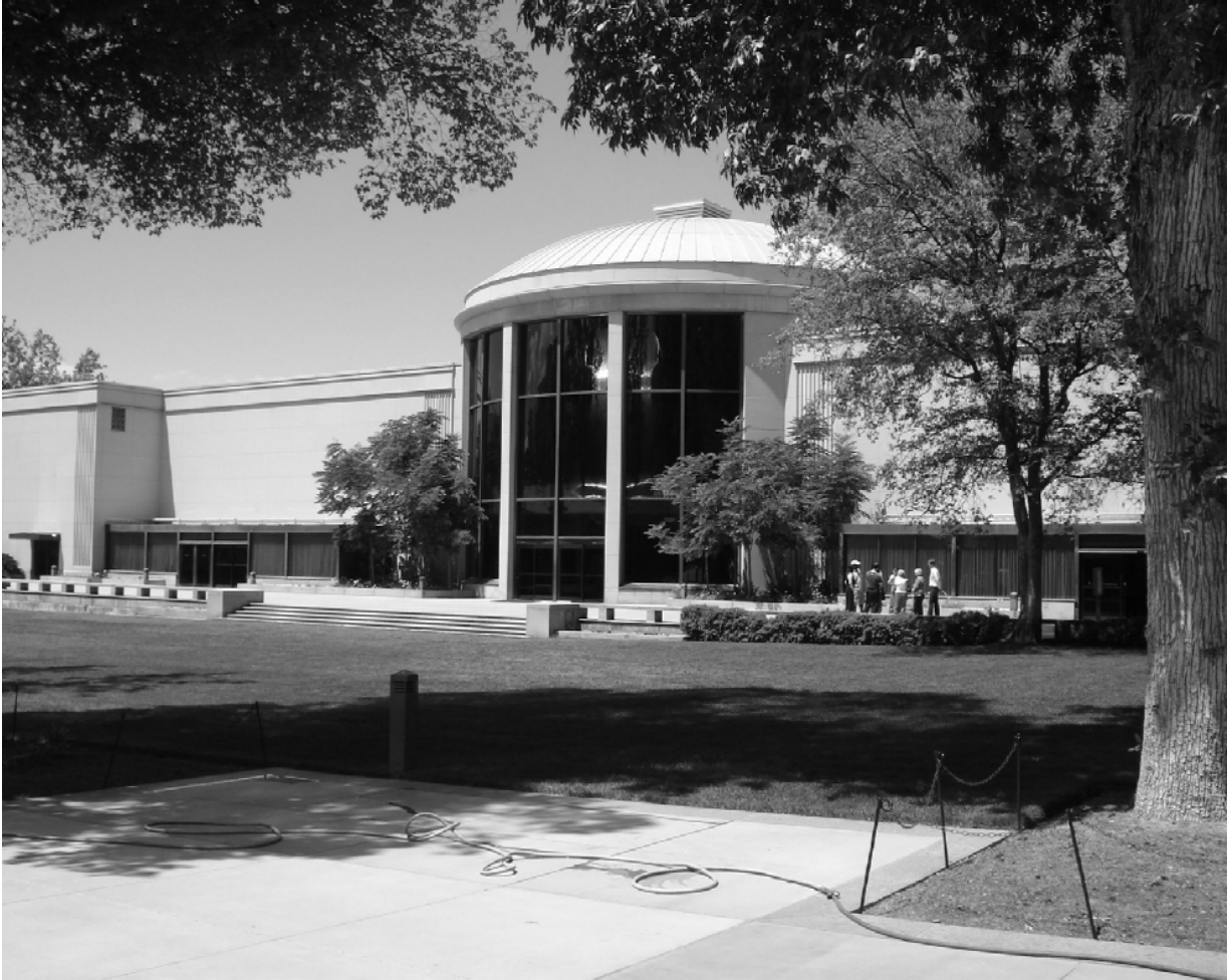
Figure 4.4: The North Visitors' Centre. Photo by author.
