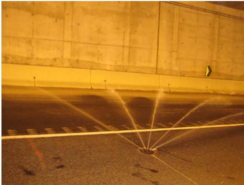
**Figure 2.1: Fixed Automated Spray Technology (FAST) Nozzle in a Hwy. 401/404 HOV Tunnel**
