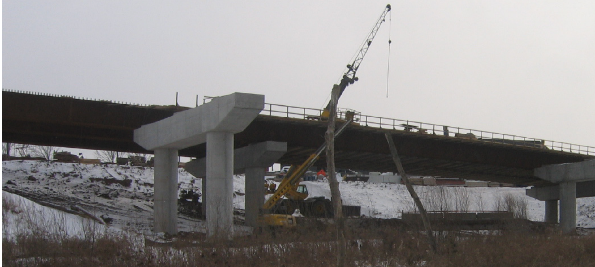
fig. 1.49 Construction of Red Hill Creek Parkway in 2006
