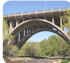
fig. 2.72 Bridging 16 Mile Creek
