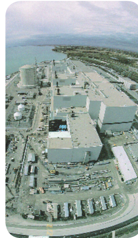
fig. 2.42 Darlington Nuclear Power Plant
