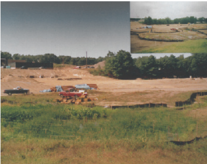
fig. 3.25 Devens Wetland Construction
