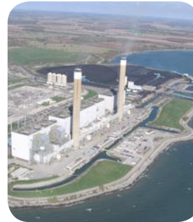
fig. 2.53 Nanticoke coal powered thermal power plant.
