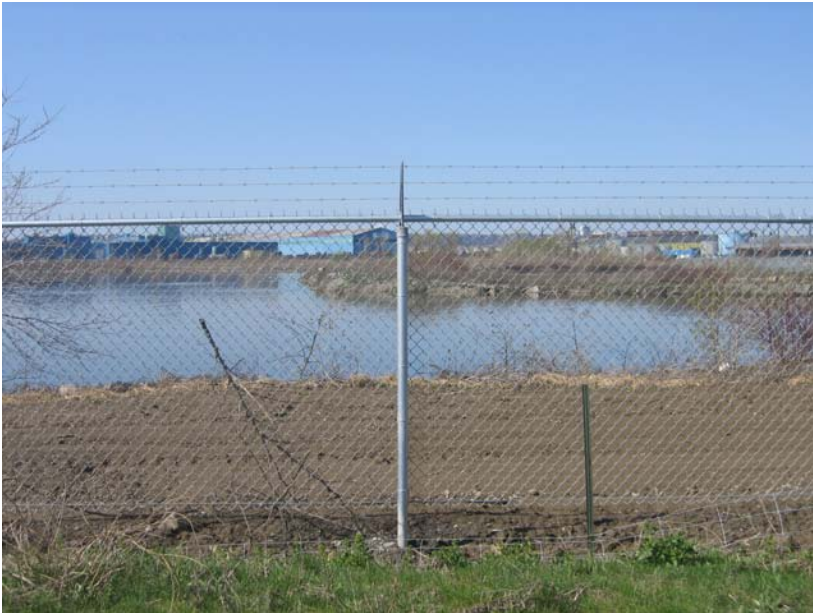
fig. 1.44 Typical fence condition separating industrial use from the open space that surrounds Windermere Basin
