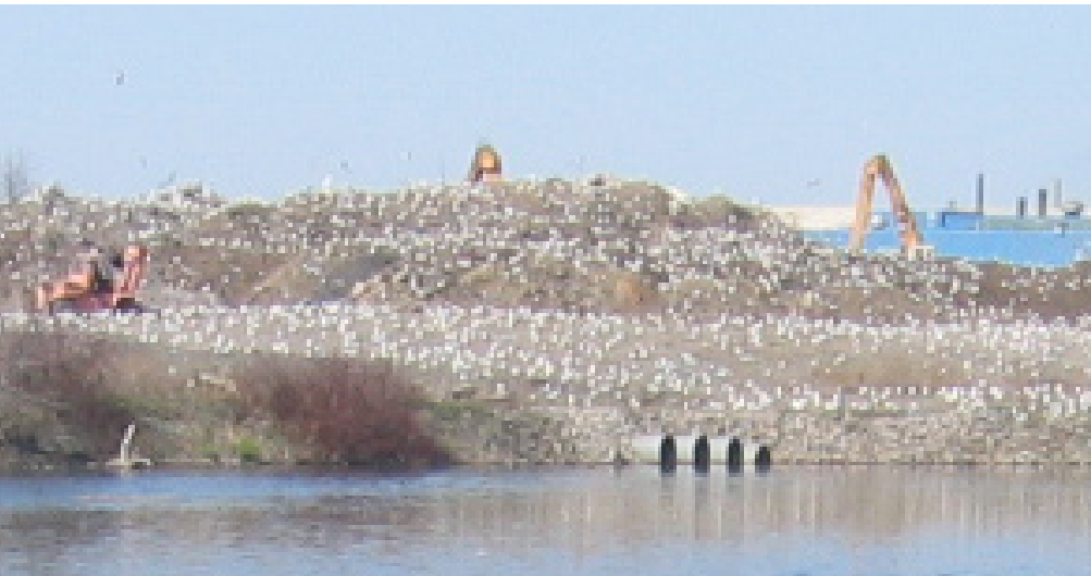
fig. 1.35 Combined sewage overflow discharge point into Windermere Basin – In a combined discharge system raw sewage is mixed with rain water. When there is a heavy backup the combined water is discharged into the environment.
