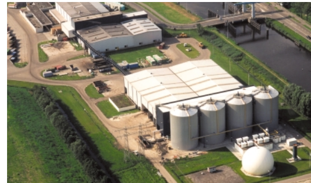
fig. a3.7 Vagron plant (Groningen) for separation and digestion of the organic fraction of MSW
