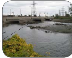
fig. 4.26 Water surfaces — a representation of prominent artificial or naturally adapted water systems
