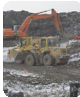
fig. 2.55 Glanbrook municipal landfill site at the head of the Red hill creek watershed.
