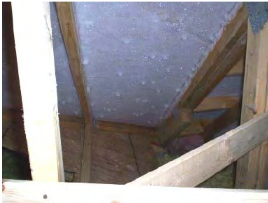
Figure 5.2 – Homeowner’s photo of heavy frost in attic
