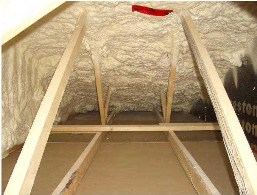
Figure 5.35 – Low-density oc-SPF and cathedralized attic inside of Roof Panel S2
