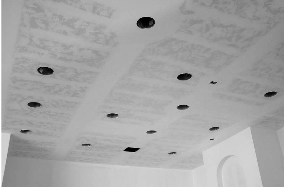
Figure 2.7 – Complex ceiling in newer house (numerous penetrations for lights and speakers)
