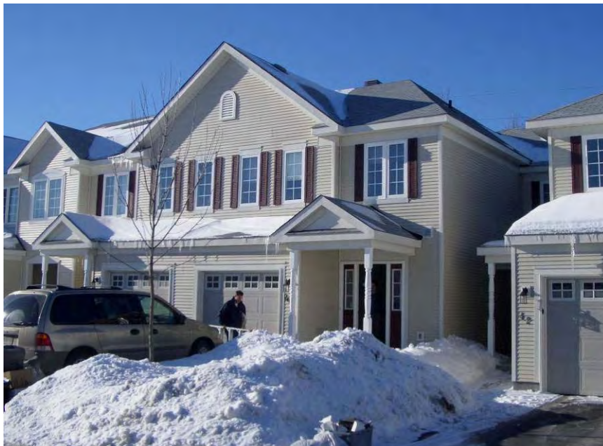
Figure 5.3 – Photo of Ottawa field investigation house
