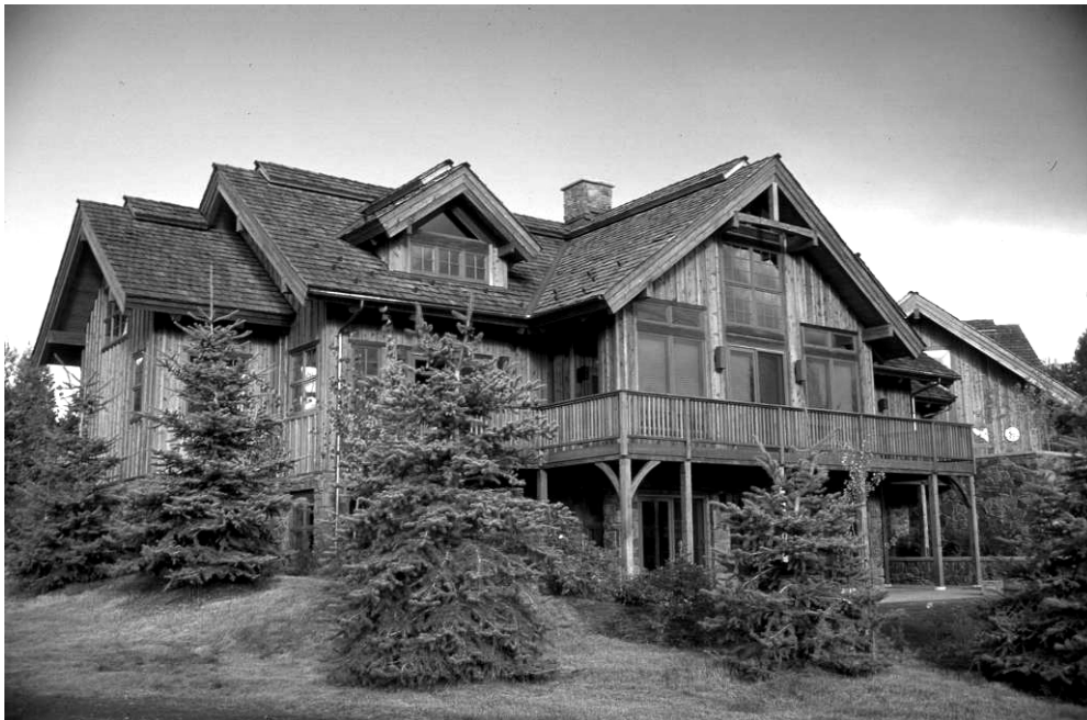
Figure 2.6 – Newer house with complex roof geometry (dormers, valleys and many ridge lines)
