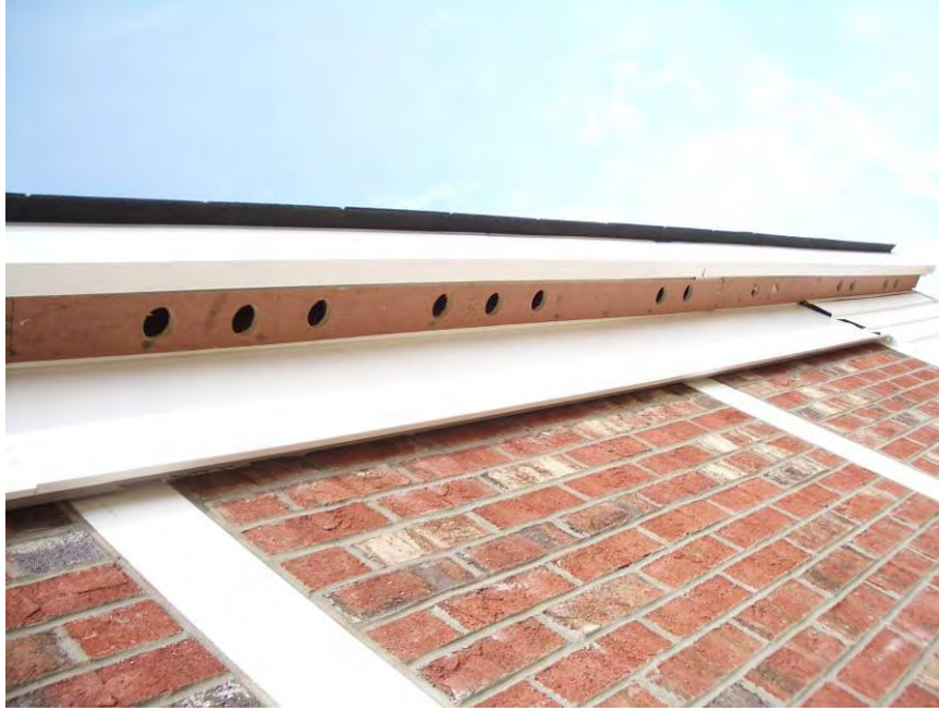
Figure 5.60 - Soffit vent openings
