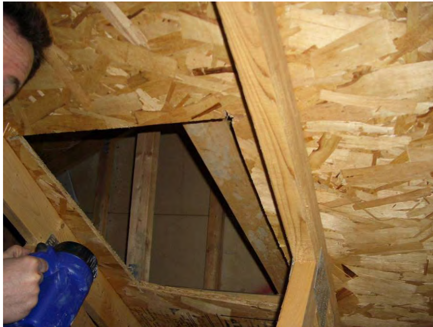
Figure 5.6 – Ventilation opening between attic compartments
