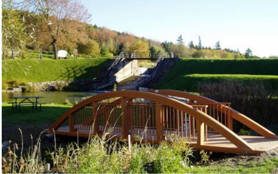
Figure 9: Bridge, located in Millbrook, Ontario, constructed using oriented wood-plastic-composite material (Everarch, 2008)
