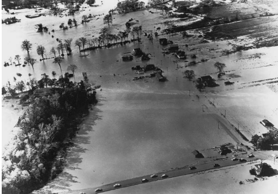
Figure 1.1-19 Flooding Caused by Hurricane Hazel 1957
