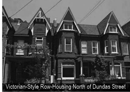
Victorian-Style Row-Housing-North of Dundas Street
