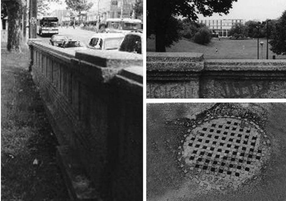
Figure 1.2-21, 1.2-22 (left & top, right) Buried Harbord Street Bridge
