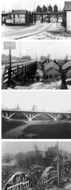
Figure 1.2-16 (top, left) Sulli Crescent Bridge (looking west toward Shaw St) Early 1900s
