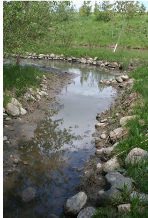
Figure 10. Critter Creek Upstream restored riffle and pool segment.
