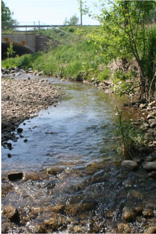
Figure 10. Forwell Creek restored riffle and pool segments.
