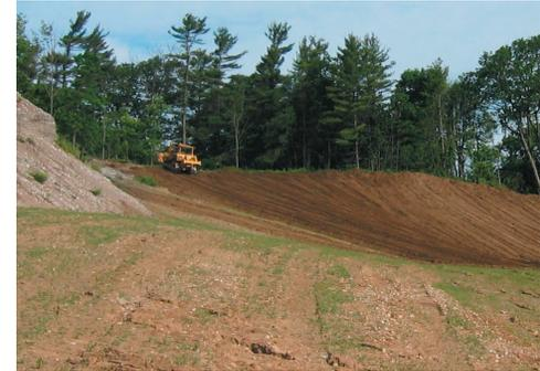
Fig. 60 | Grading banks to a 3:1 slope
