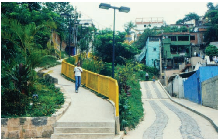
FIGURE A.13 Aerial view of Fernao Cardim favela-bairro in Brazil; some of the major upgrading projects implemented in this community are: the construction safer and cleaner pedestrian pathways; building retaining walls and bridges along and across the river.
