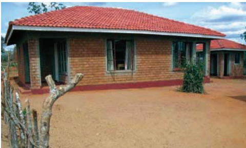
FIGURE A.40-46 Images of the construction of the Nyumbani Village. Construction labour for the village was mostly done by member of the surrounding community.
