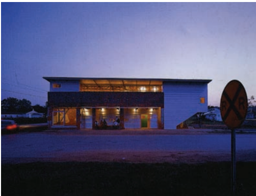
FIGURE A.8-9 TOP LEFT: The Bryant (Hay Bale) House in 1994. TOP RIGHT: The changes the house has adapted over time (2000).
