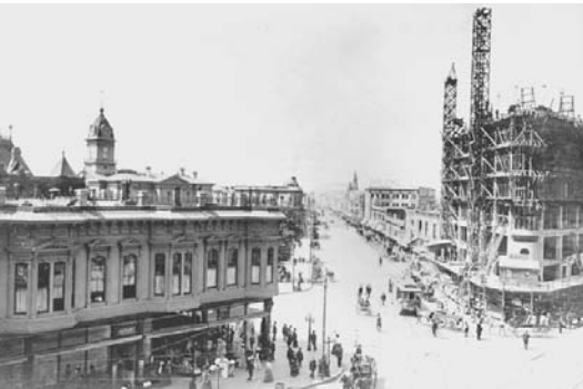
1.6 Major Construction - Broadway & San Pablo (1906)
