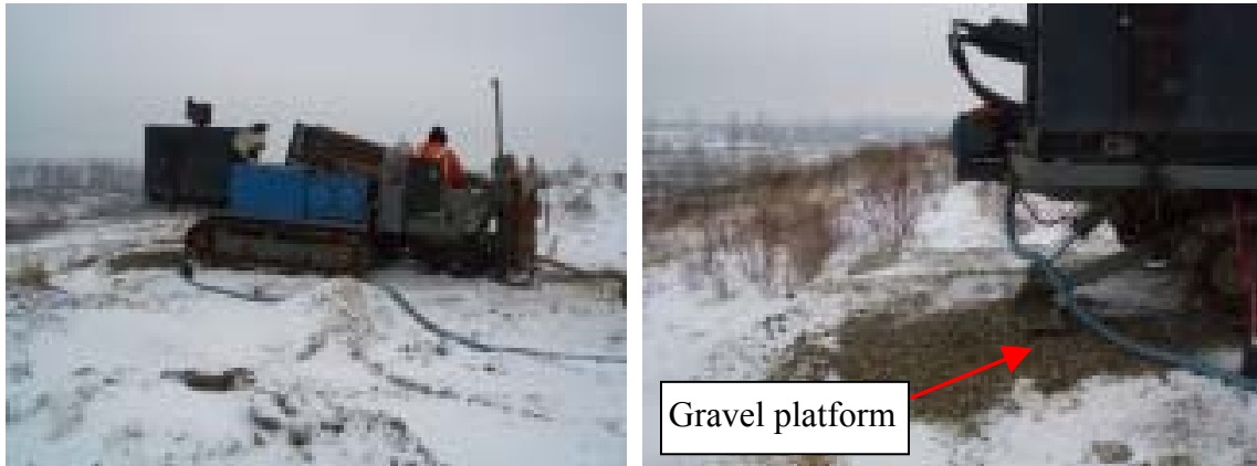
Figure 6-21: Drill Rig Sitting for West Well Installation
