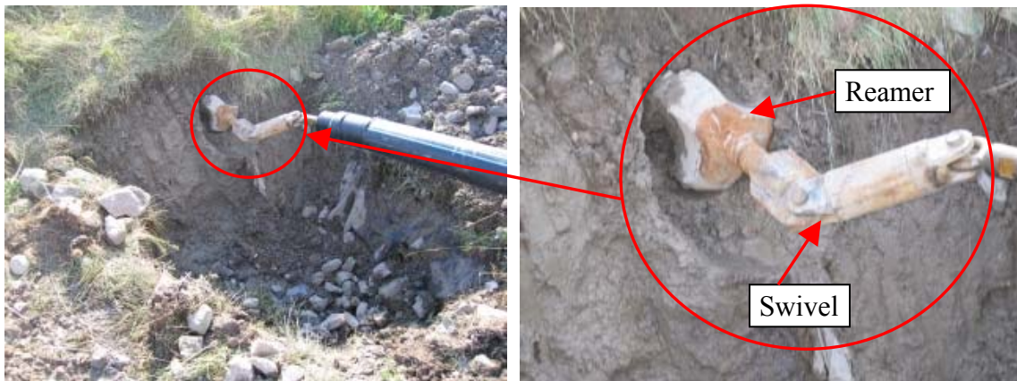
Figure 6-7: The entering of the 305 mm Reamer into the Bore during Pullback
