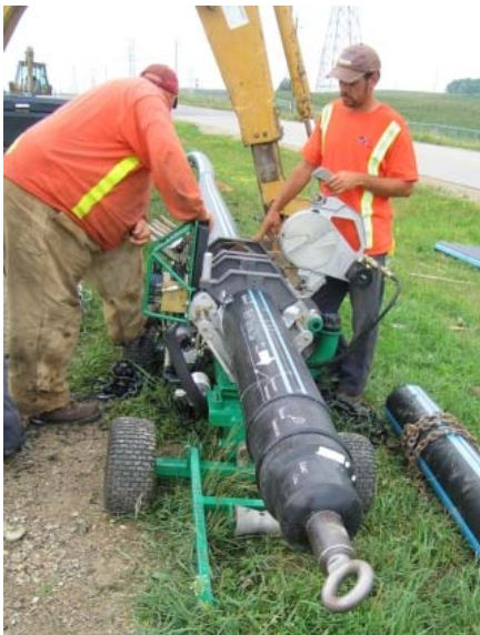
Figure 6-6: Fusion of Instrumented Test Section onto the 200mm Carrier Casing.
