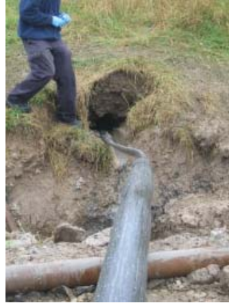
Figure 6-18: Reduced Diameter in 100-mm Perforated Pipe after Last Attempt
