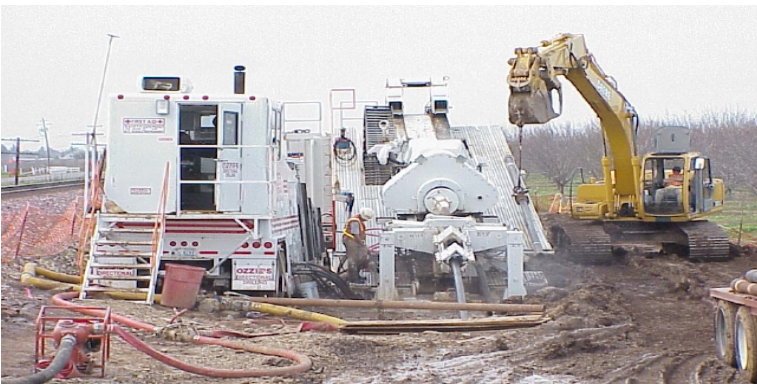
Figure 3-5: Maxi-HDD Rig (HDD Consortium 2001)
