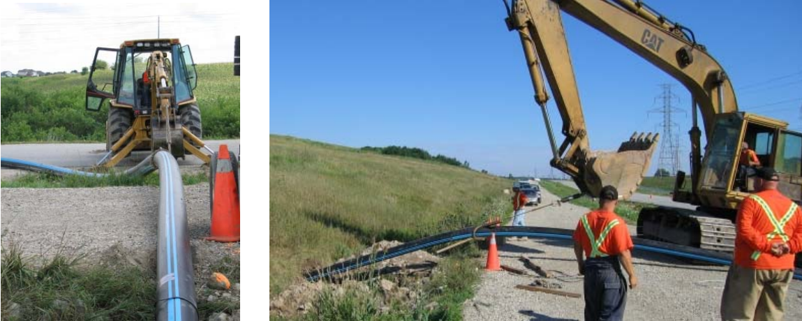
Figure 6-8: Pullout of Carrier Casing during 1 st Pullback Attempt by Backhoe & Excavator
