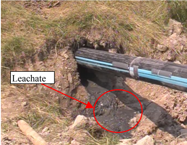
Figure 6-11: Leachate Flow during 2 nd Pullback of 200-mm HDPE Casing
