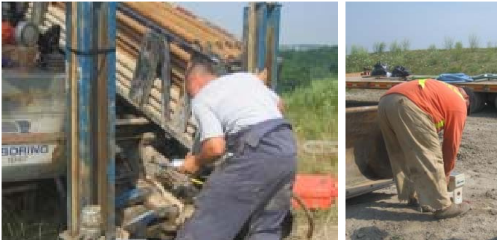
Figure 6-3: The Combination of Wireline System and Walkover System.
