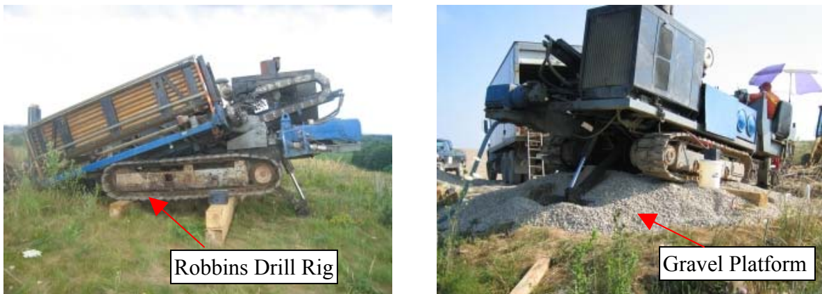
Figure 6-2: The Addition of Gravel Platform for Drill Rig Stability
