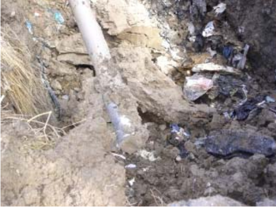
Figure 6-22: Drill Head Breakthrough Condition Upon From West Well Pilot Bore
