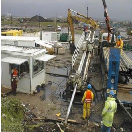
Figure 4-1: HDD Horizontal Well Construction at the Rainham Landfill (Cox et al 2000)
