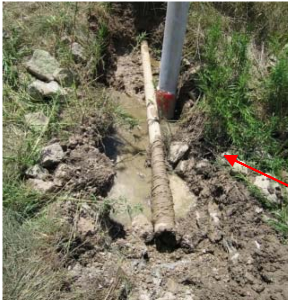
Figure 6-5: Breakthrough of pilot boring
