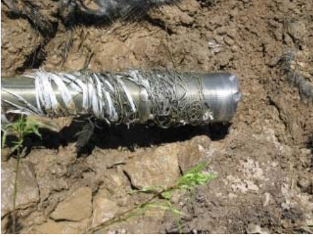
Figure 6-4: Drill Head used for the East Well installation
