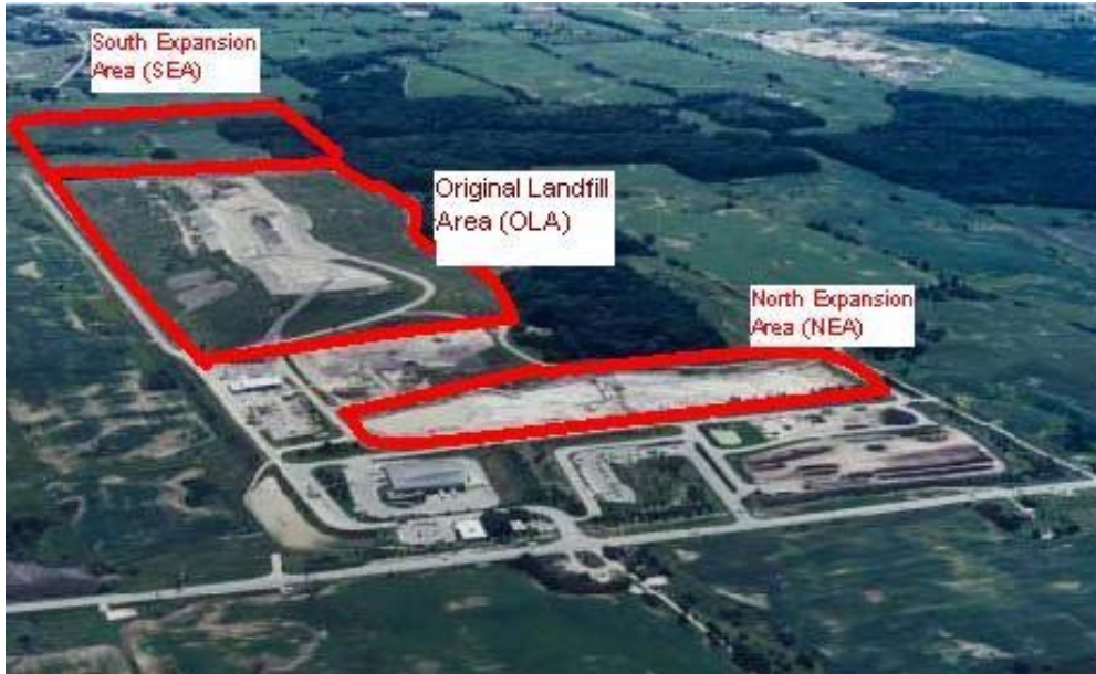
Figure 2-2: Waterloo Landfill Site (Region of Waterloo 2001)
