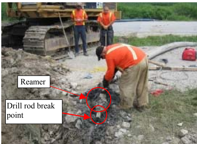
Figure 6-9: The Removal of Reamer after 1 st Pullback Attempt (July 28, 2005)
