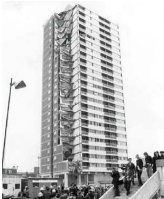
Figure 1.1: Ronan Point Apartment Building 1968 (© Daily Telegraph, 1968)
