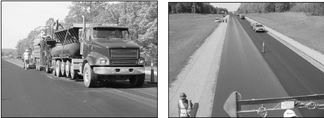
Figure 2.43: Example of microsurfacing placement [Galehouse NDA]
