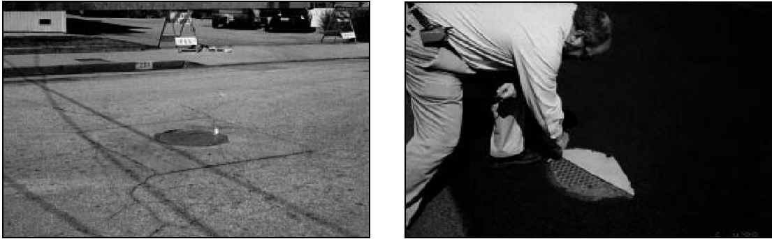
Figure 2.36: Photographs illustrating covering utilities with paper and removal after curing [Caltrans 03]
