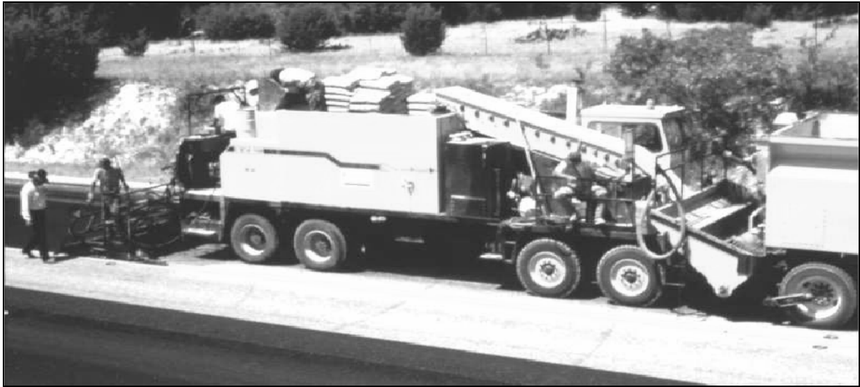
Figure 2.33: Continuous application microsurfacing placement machine [Galehouse NDA]
