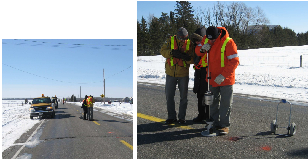
FIGURE 3-14 PFWD Testing Tutorial on the NE Experimental Site (Hwy 569, March 8, 2007)
