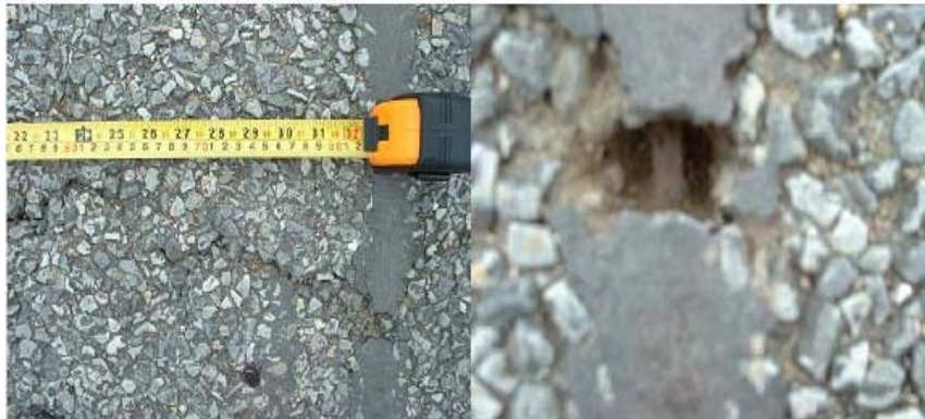
Figure 3.5: A Longitudinal Crack Crossing the Sensors
