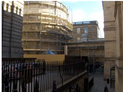
Figure 5.4: Scottish Family History Centre Under Construction, 2005
