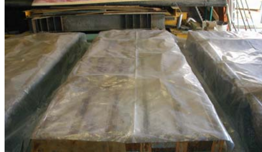
Concrete curing
