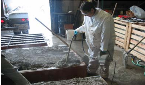
Concrete placing process
