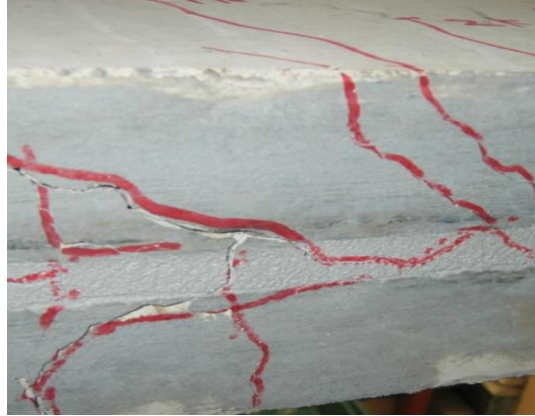
Figure 5.3: Shear cracks along the NSM groove
