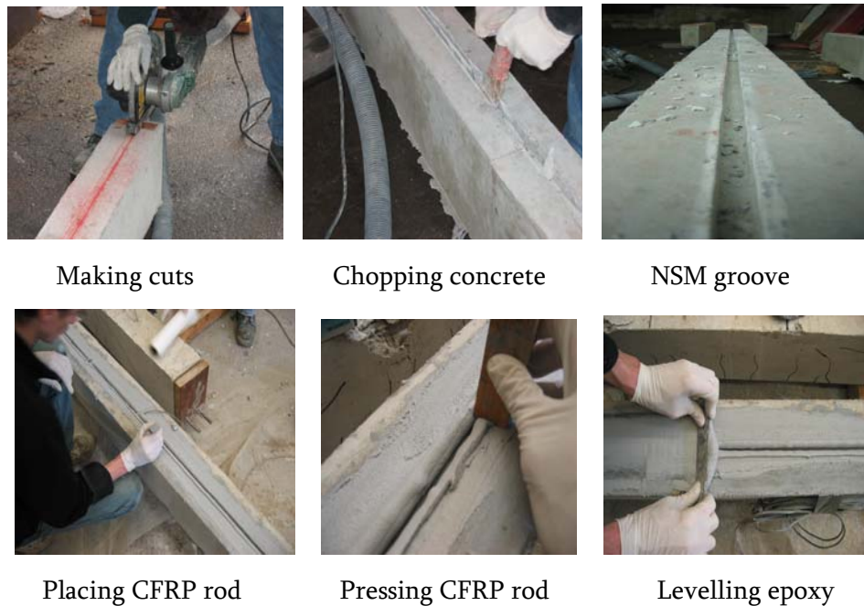
Figure 3.3: NSM CFRP application process
