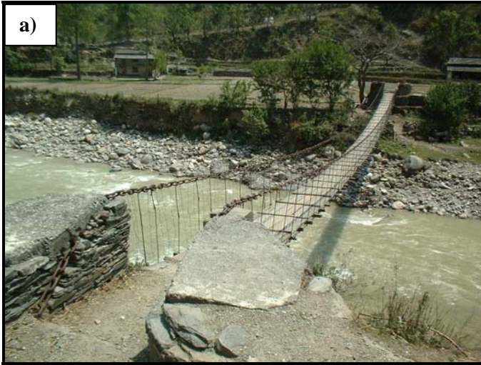
Figure 3-4: Traditional trail-bridges and river crossing means; a) An iron chain bridge, b) A primitive and risky bamboo bridge, c) A primitive and risky cable crossing, and d) A traditional dugout ferry-boat crossing
