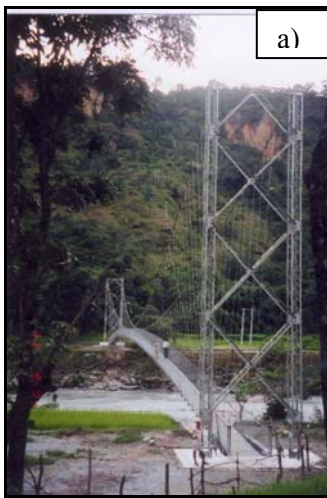
Figure 3-6: Pedestrian trail bridge types a) Suspension type, and b) Suspended type
