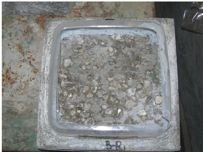
Figure 4-35, R 1 Concrete slab used for salt scaling test after 55 freeze-thaw cycles.
