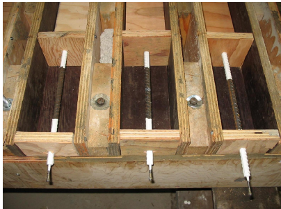
Figure 3-9, Moulds with rebars in place.
