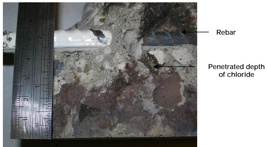
Figure 4-26, The depth of penetrated chloride in NC-RCA concrete after 165 days.
