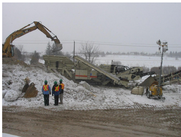
Figure 3-2, Crushing machine was used for manufacturing NC-RCA.
