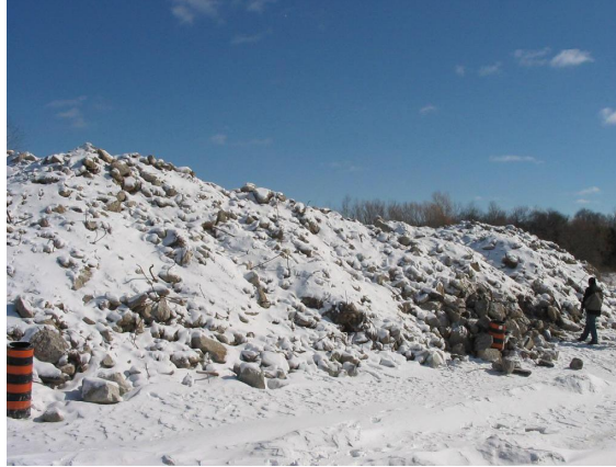
Figure 3-3, Stock-pile of demolished concrete from the bridge.
