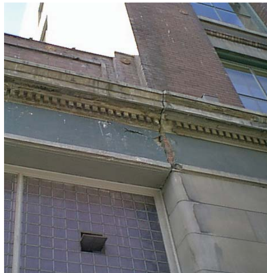
31. Human pelvis. 32. Rounded corners in tree branches. 33. Stress localization and corner cracking.
