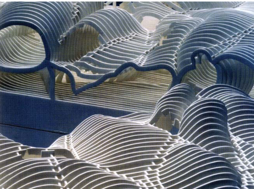
48. NOX: Structural ribs defining a doubly-curved surface are clad in narrow wood strips that follow the curvature much like in shipbuilding.
