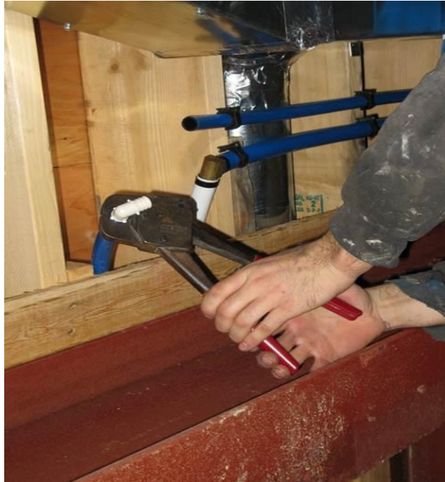
Figure #2 Manual crimper
