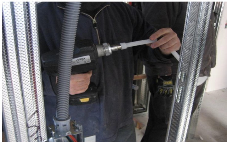
Figure #5 Flexible Piping Stretching Tool
