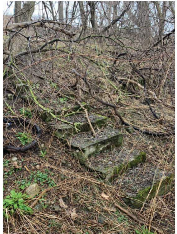
Figure 6: Image of stairs remaining from the demolition of several houses by the GRCA Paris, Ontario. 2023, Photo by author.
