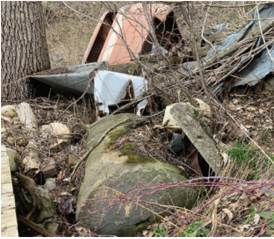
Figure 9: Car frame, twisted metal, and column shaft, Paris, Ontario. 2023, Photo by the author.
