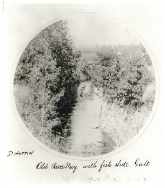
Figure 30: D. Herriot, Image showing an 'old' raceway and 'fish slide'. Courtesy of the Cambridge City Archives.
