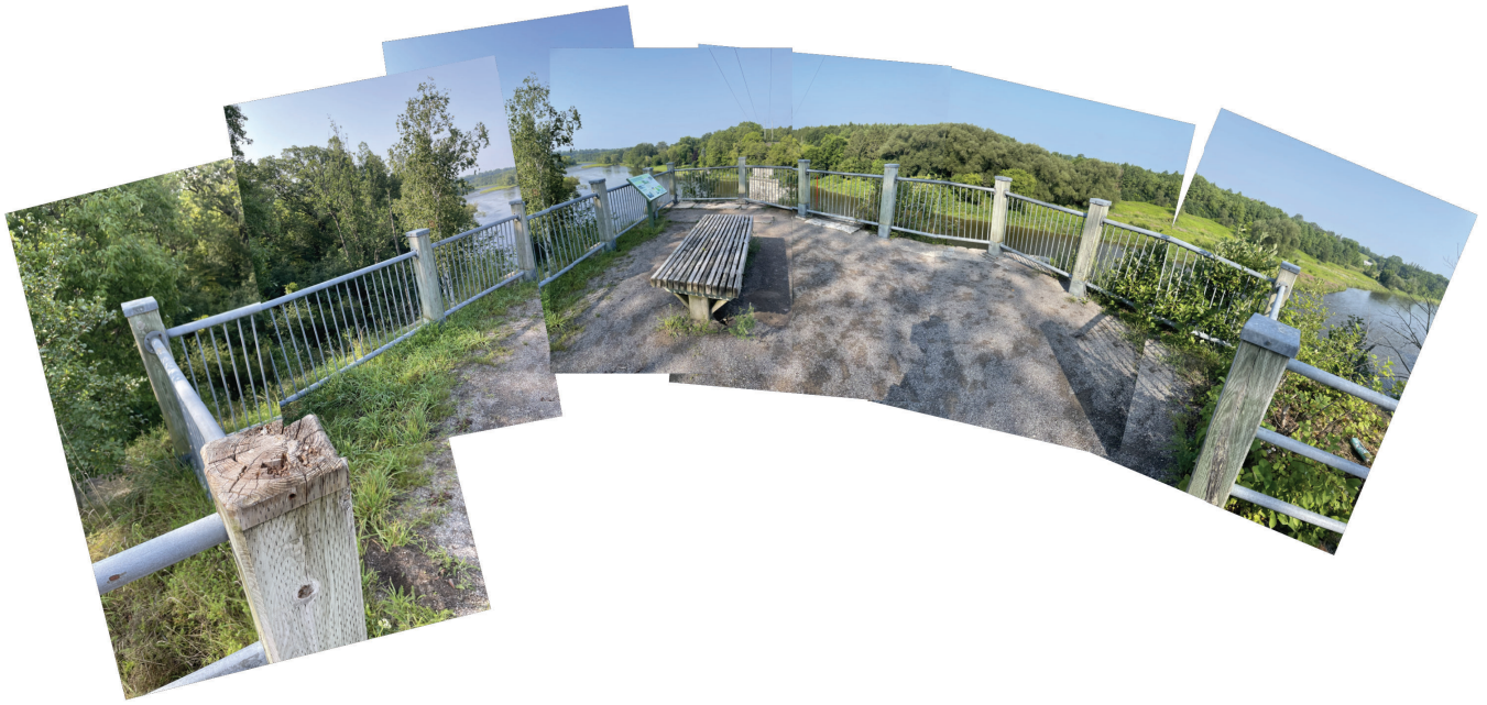
Figure 60: Composite image of the existing lookout at the Great Western Railway bridge abutments near Paris, Ontario. 2023, Photo by author.
