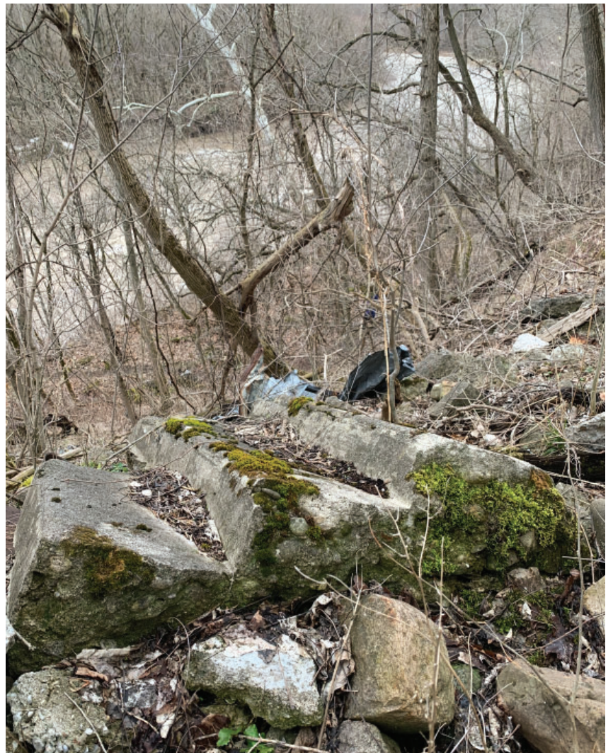
Figure 7: Image of stairs remaining from the demolition of several houses by the GRCA Paris, Ontario. 2023, Photo by the author.
