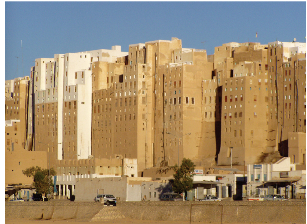
Fig. 1.3 Five to nine stories, the mud buildings of Shibam are described as the oldest skyscrapers in the world, since some of the buildings are five hundred years or older. Obviously, given the non durable nature of the construction material, all the buildings need to be regularly renovated.
