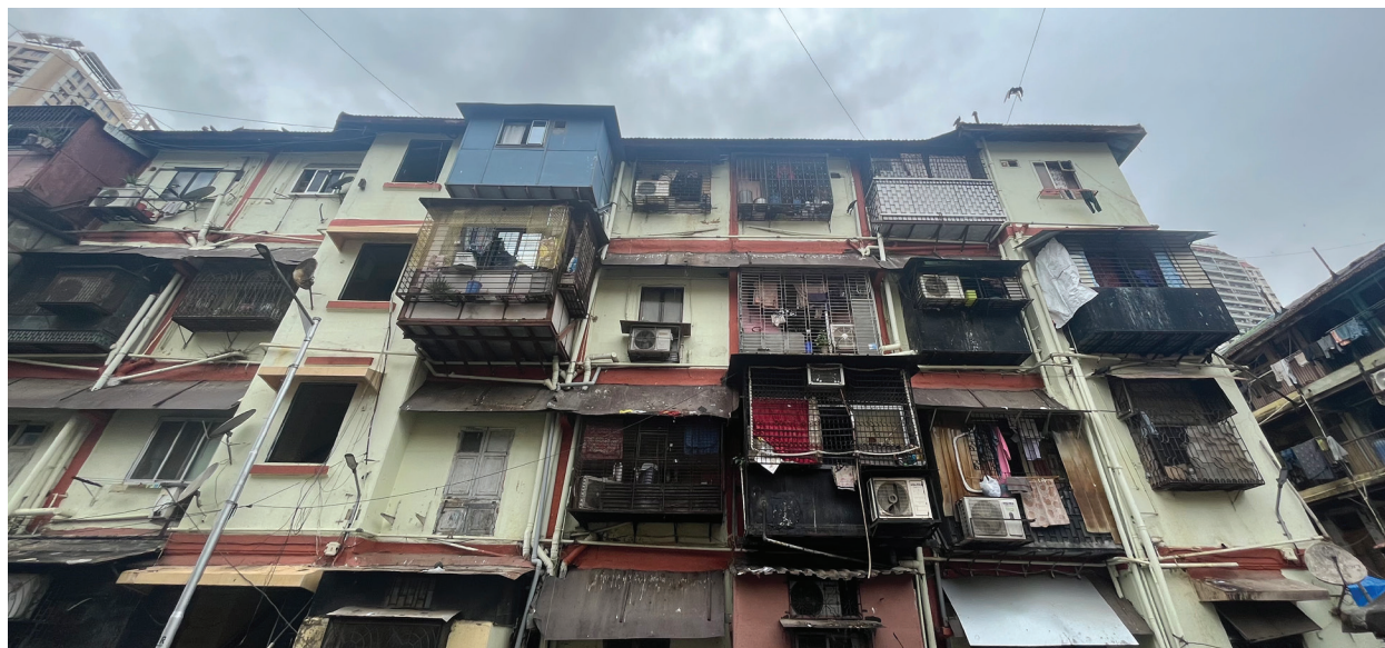
Fig. 4.30 Facade with its extensions and modifications BIT Chawls
