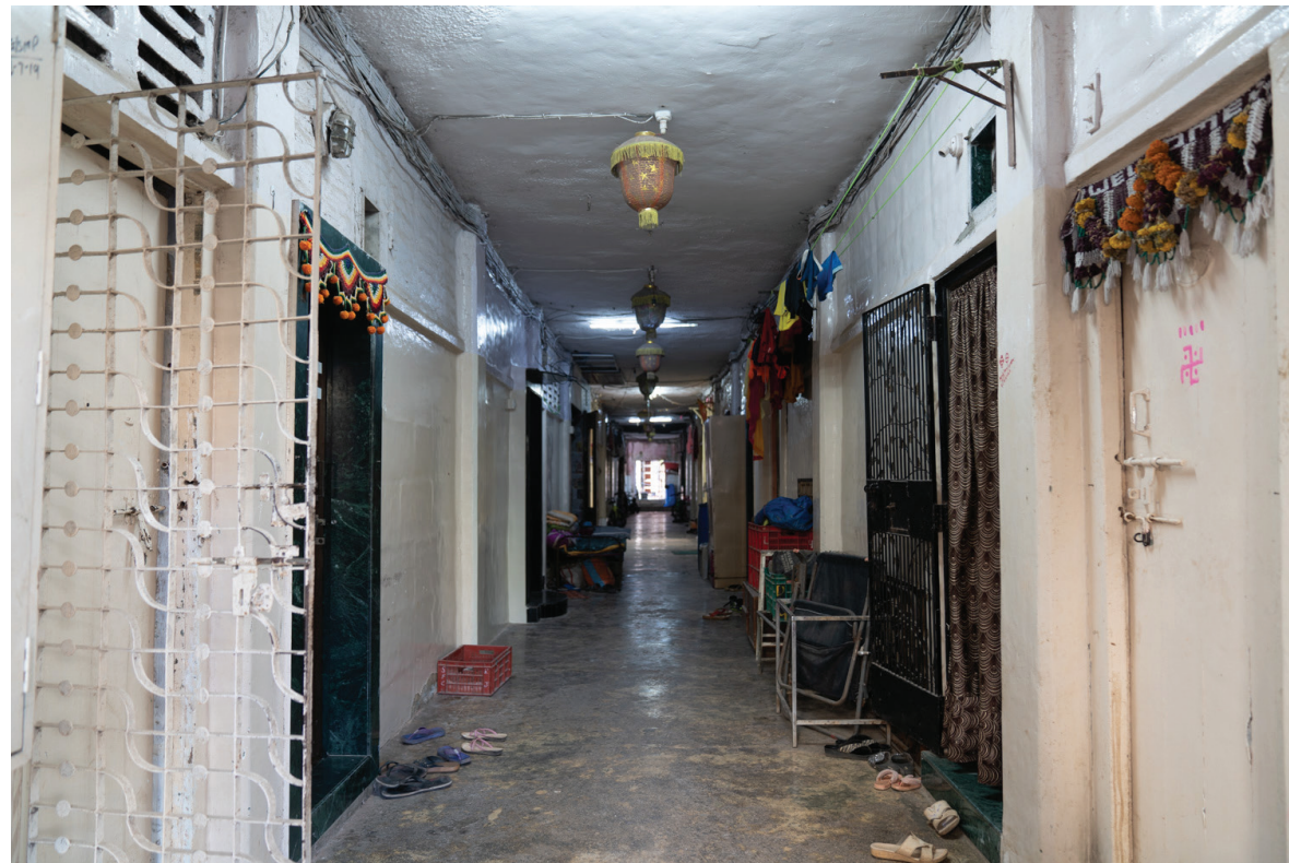
Fig. 5.34 Upper floor corridor
