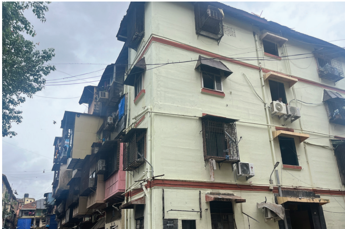
Fig. 4.27 Corner of BIT Chawl building
