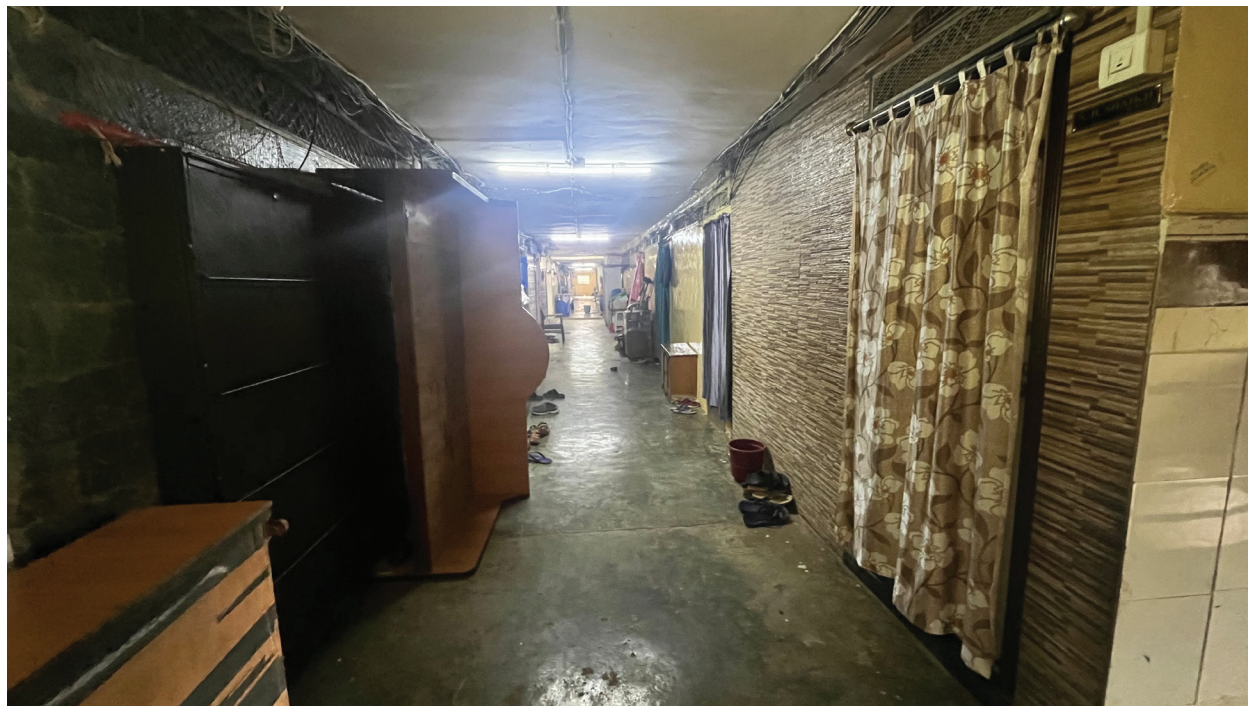
Fig. 4.33 Corridor with furniture spill out BIT Chawl
