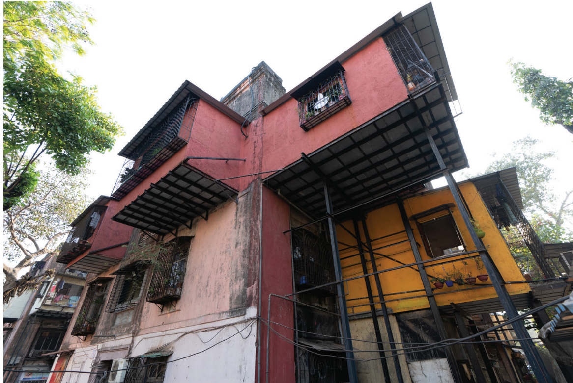
Fig. 5.23 Residential Extension Corner Unit 3
