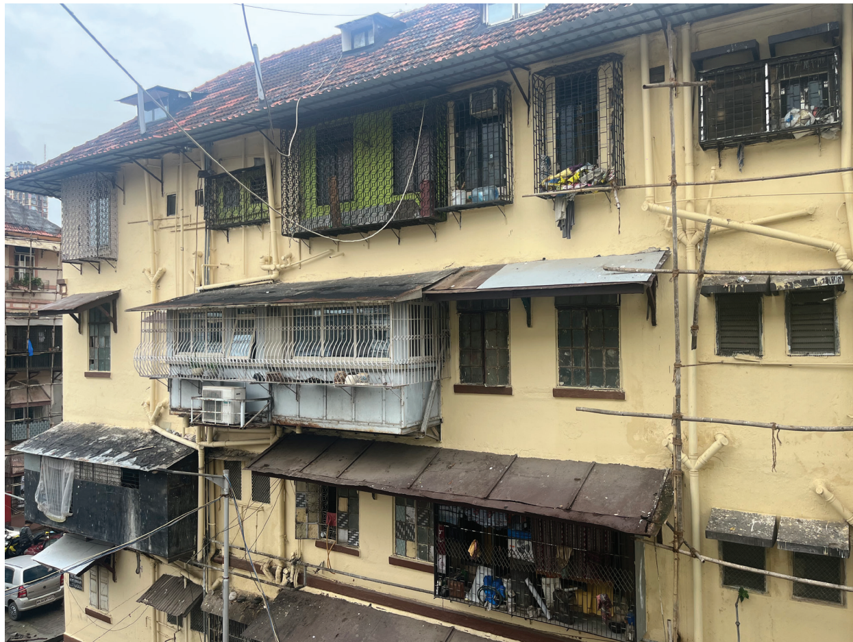
Fig. 4.29 Facade with extensions and personalisations BIT Chawls
