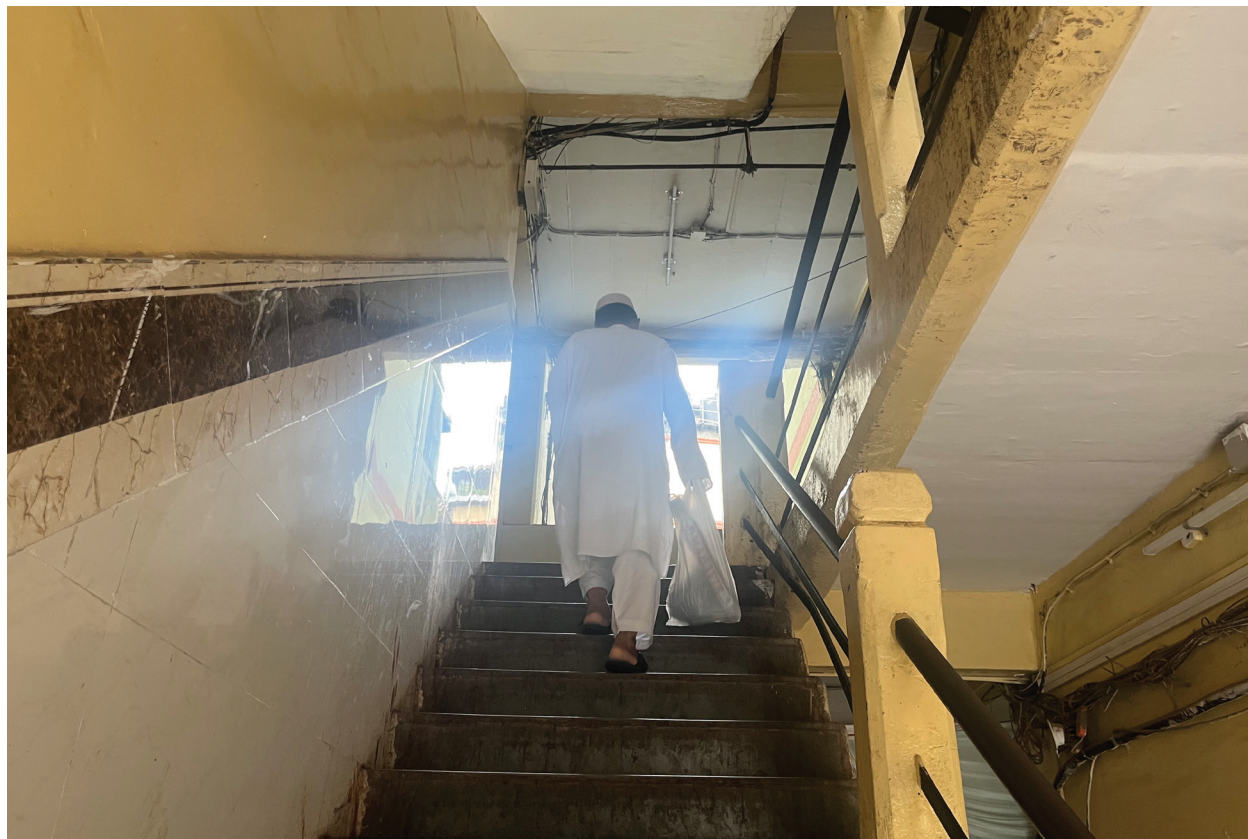
Fig. 4.36 Stairs BIT Chawls
