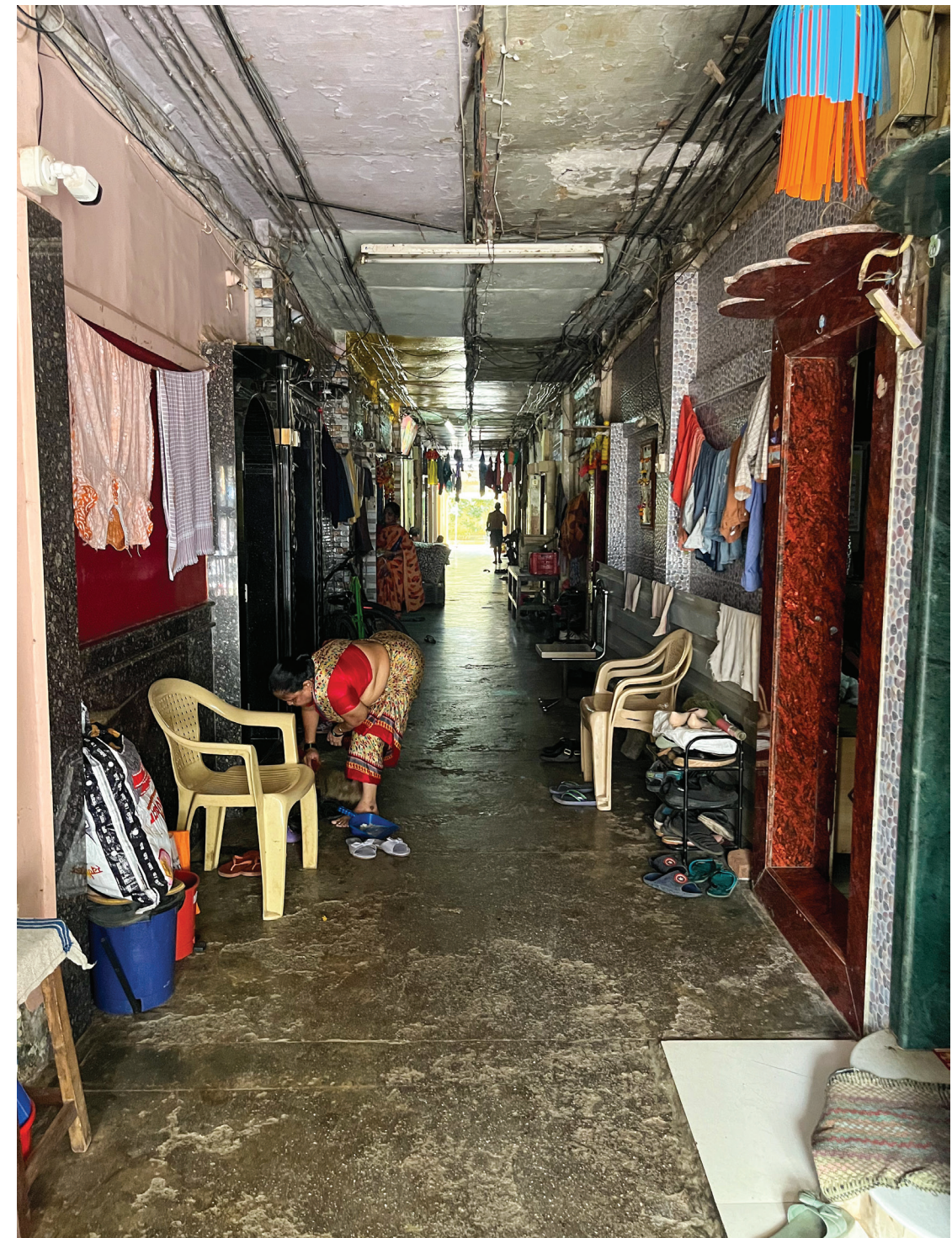
Fig. 5.35 Ground floor corridor
