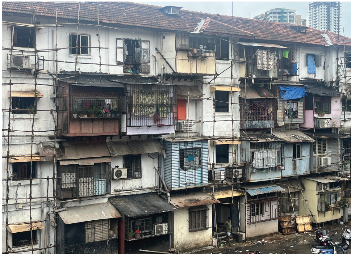
Fig. 4.26 Extensions from facade BIT Chawls
