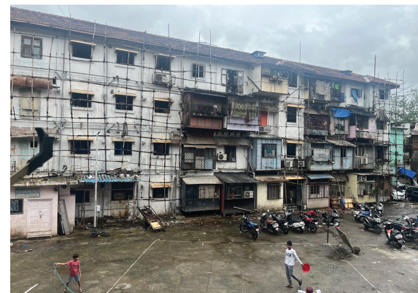
Fig. 4.25 Facade under repairs BIT Chawls
