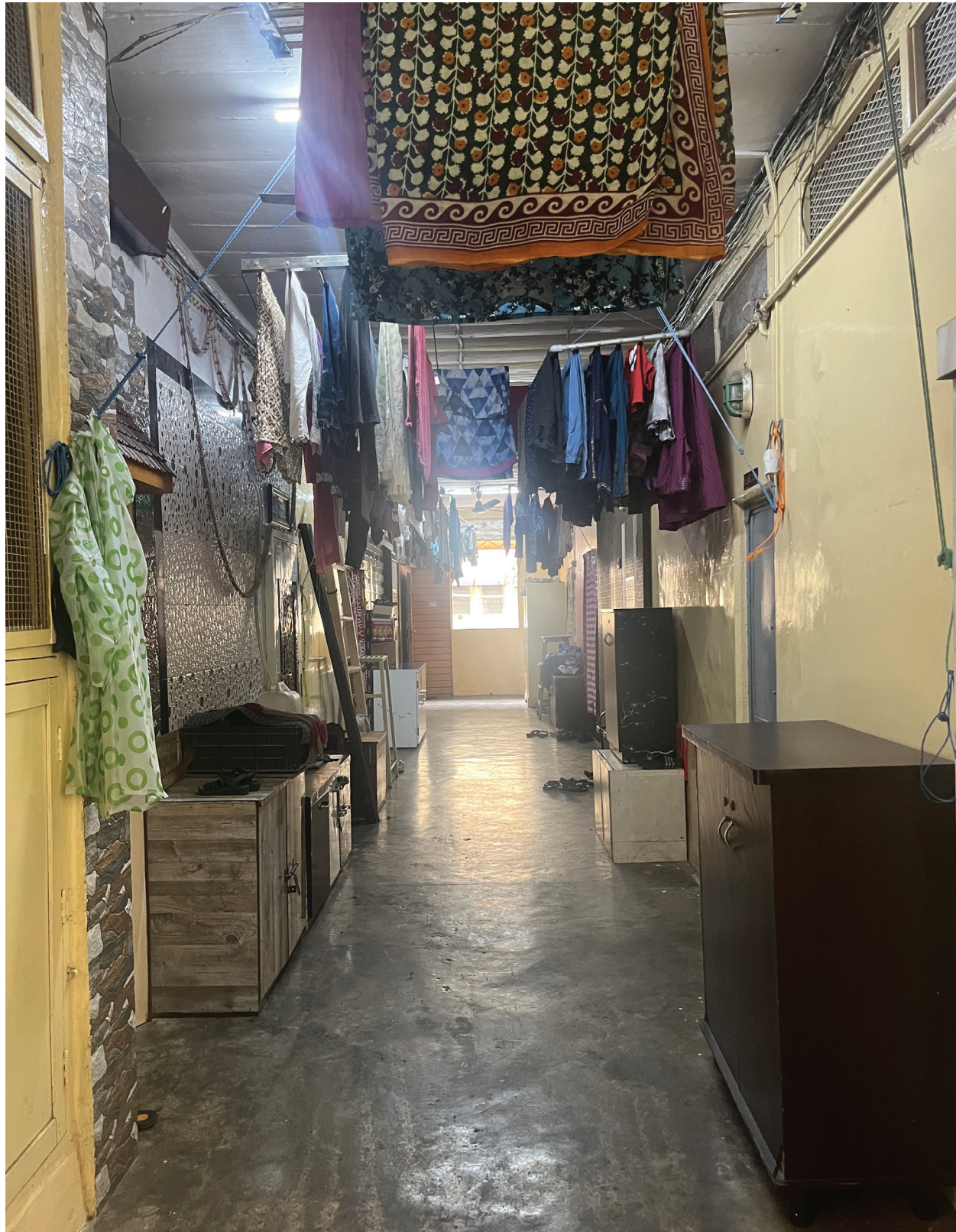
Fig. 4.38 Corridor with window at the end BIT Chawls.
