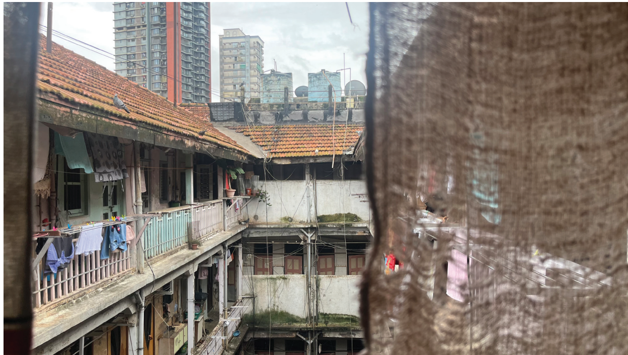
Fig. 4.14 Bhatia Chawl courtyard with high rises in background
