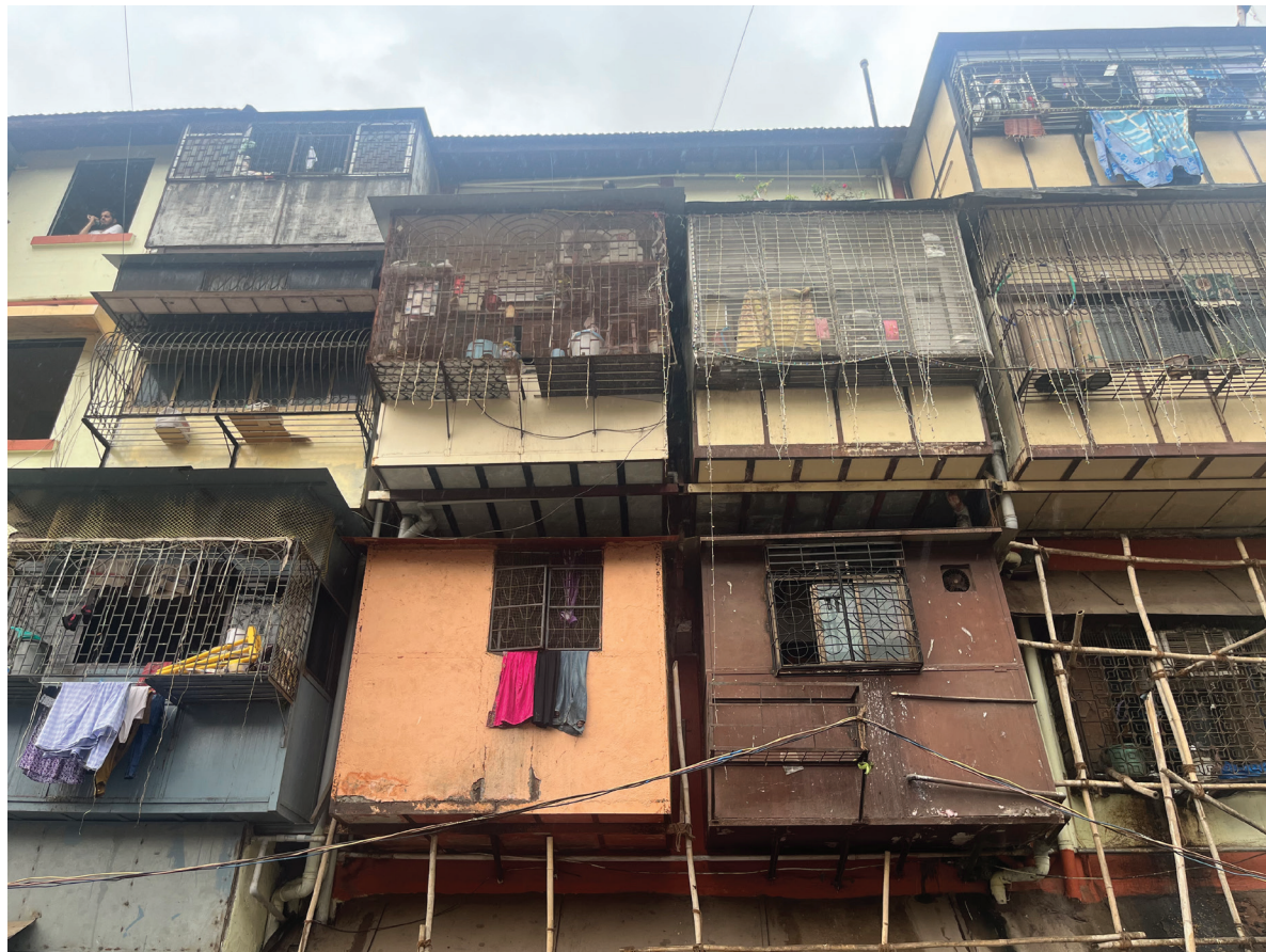
Fig. 4.42 Scaffolding and extensions BIT Chawls
