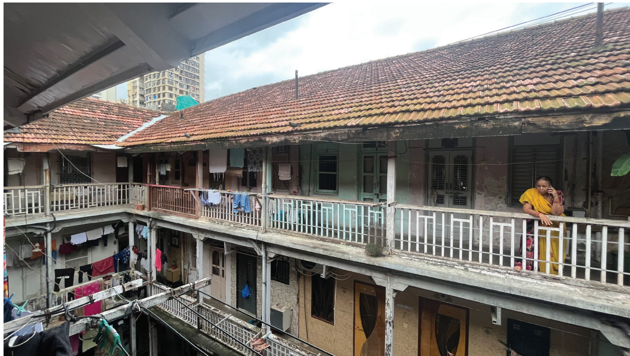
Fig. 4.15 Courtyard and Roof Bhatia Chawls
