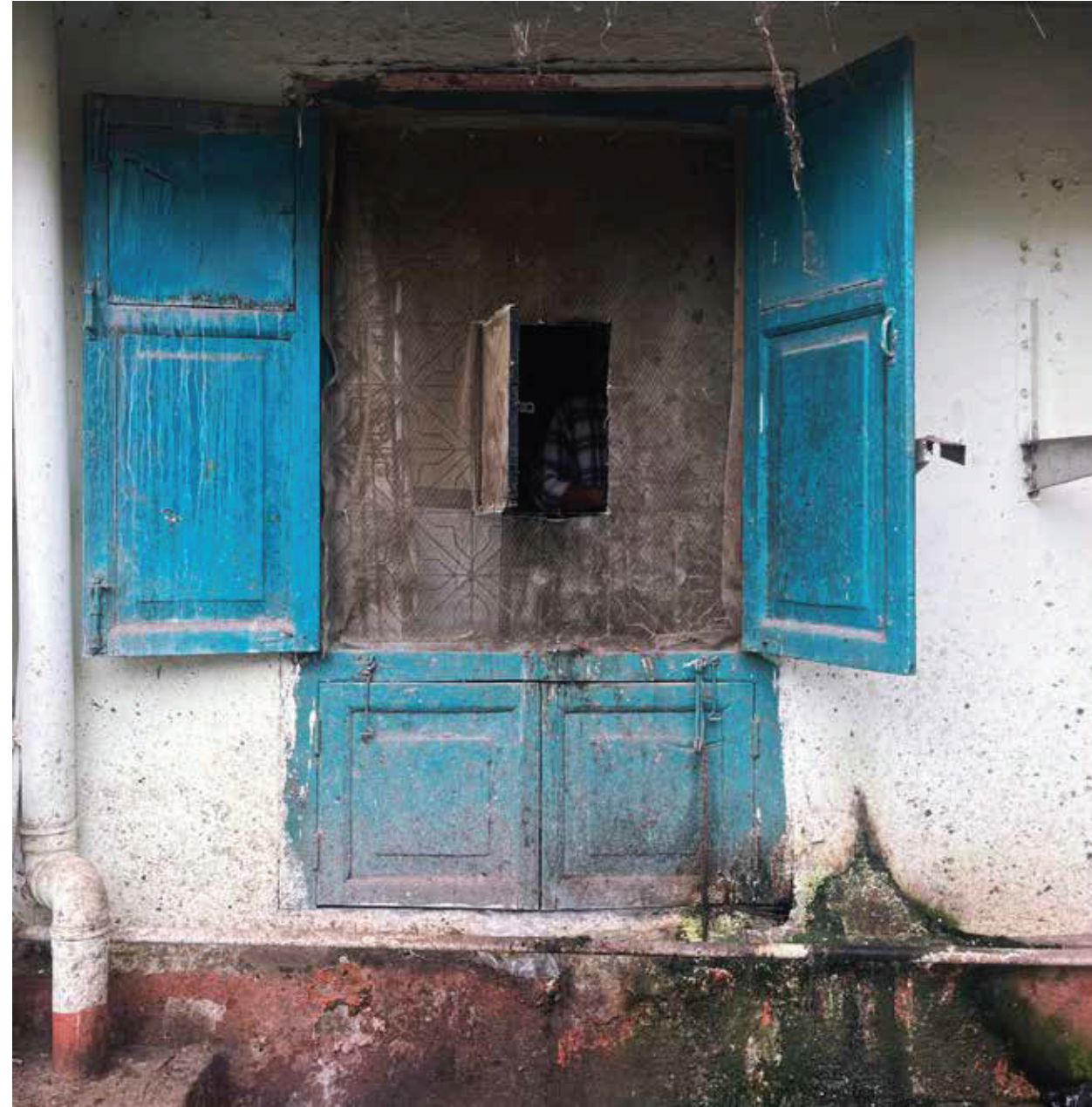
Fig. 1.14 A smaller window inside a window: Original wooden window on a weathered building, modified to add a security metal grill, a mosquito net attached with zipties for protection against insects, and a small, functional opening in the grill for accessibility.
