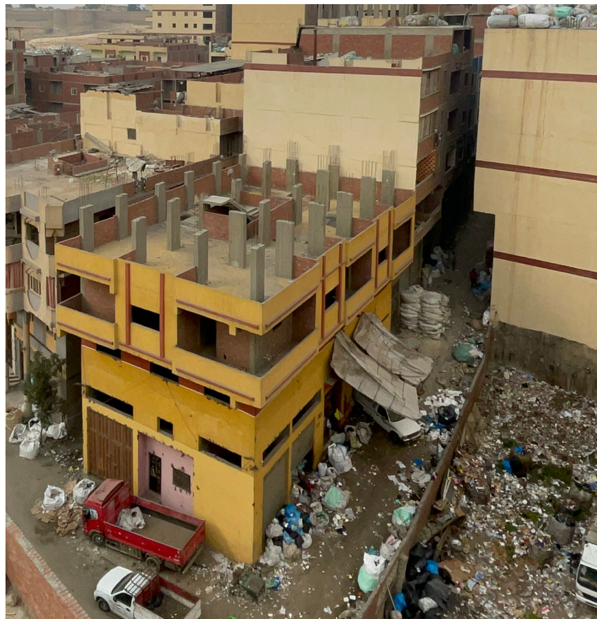
Fig.5.19 An informal building typology with exposed structure and rebar. Manshiyat Nasser, Cairo. Photographed by author
