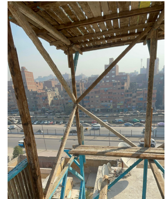
Fig.7.5 Pigeon Tower Structure.
