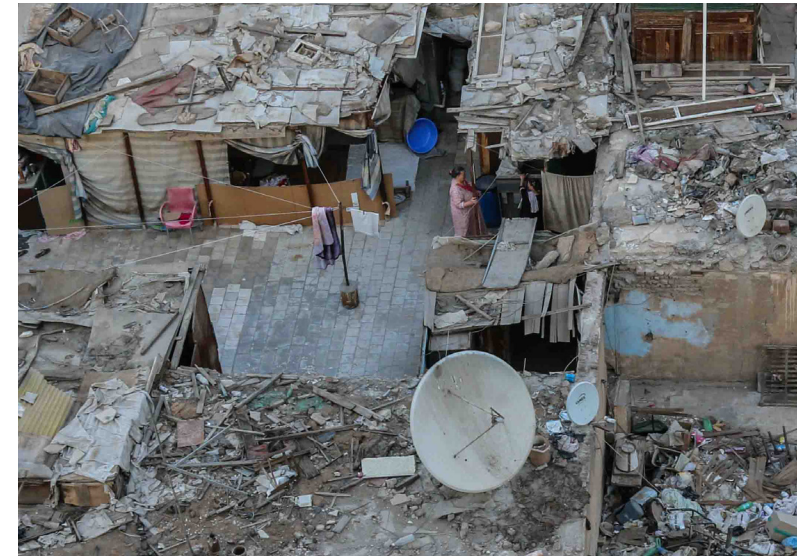
Fig.5.3 View of the roof terrace of a building in Mouinra district. Several families share the terrace together. By Marie Piessat
