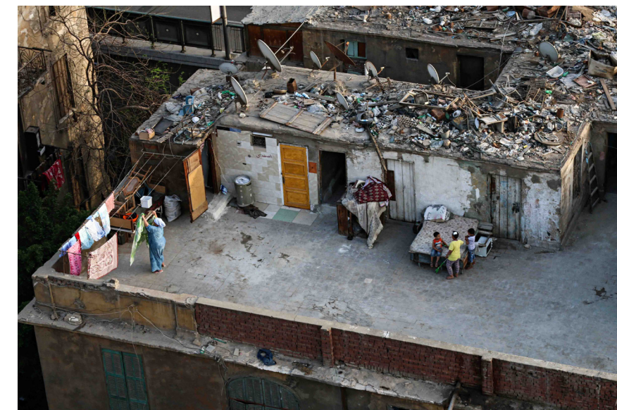
Fig.3.28 View of a family's home in Boulaq. The roof terrace offers a safer playground for children than the street. Photographed by Marie Piessat, April 2017
