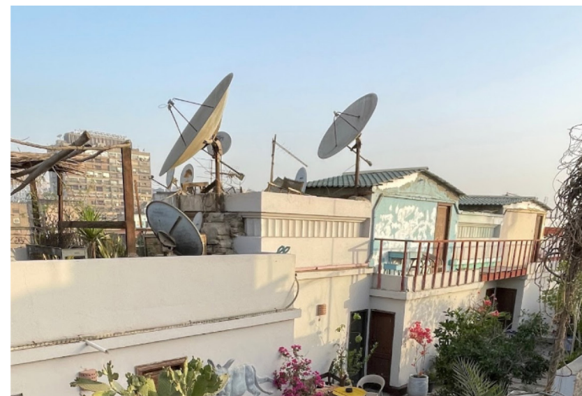
Fig.5.48 A view of the second floor of Dahab Hostel with Satellite Dishes. Photographed by owner
