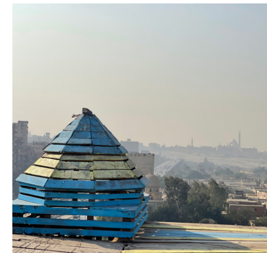
Fig.7.11 View from the top of the Pigeon loft showing the Citadel and Historic Cairo
