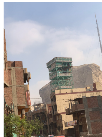
Fig.7.17 Street View of the entrance of Manshiyat Nasser showing Pigeon tower on rooftop
