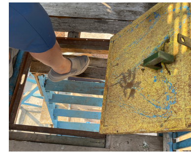
Fig.7.14 A trapdoor to access the Pigeon Loft
