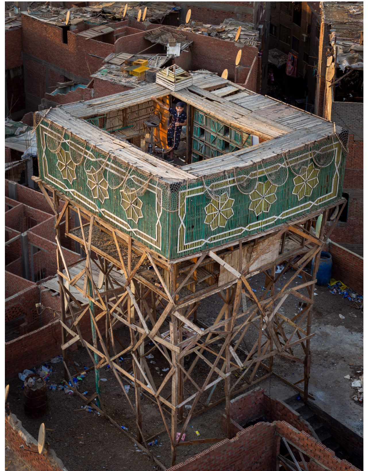
Fig.5.12 Pigeon Tower in Manshiyat Nasser. Photographed by Andreas Trenker
