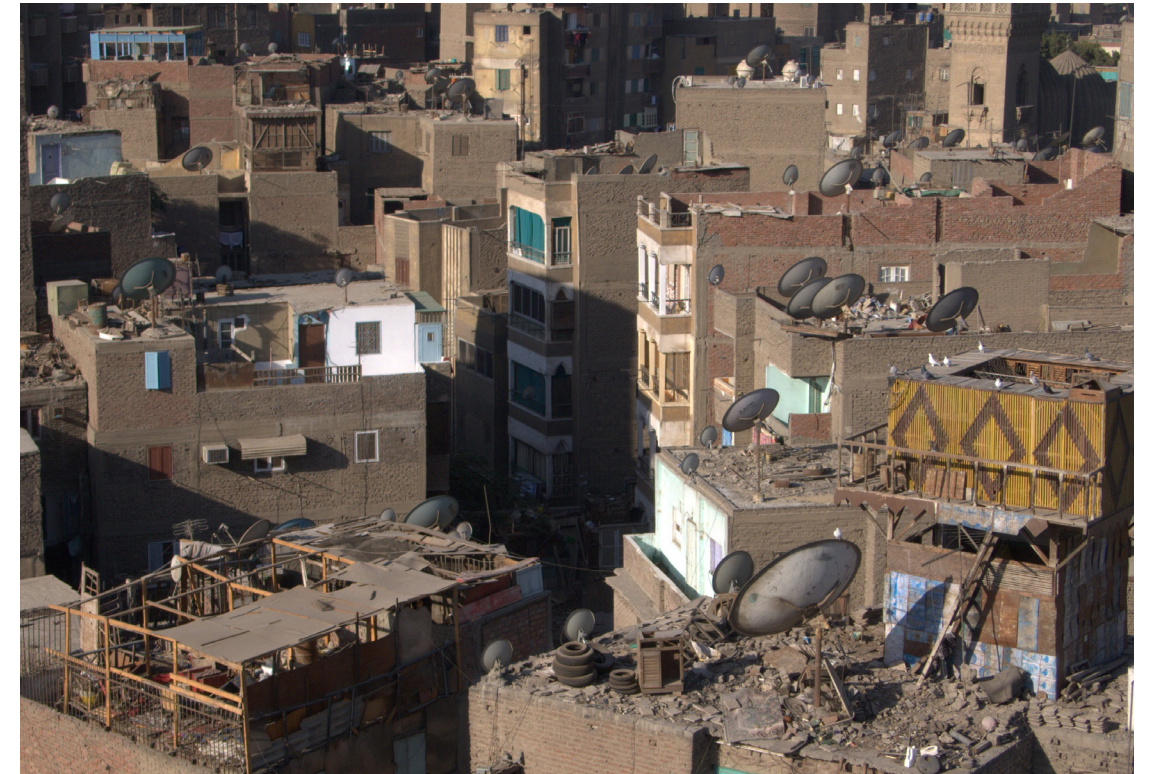
Fig.3.2 A view of the rooftops in 'Islamic' Cairo with the typical clustering of satellite dishes. Jason L, Flickr
