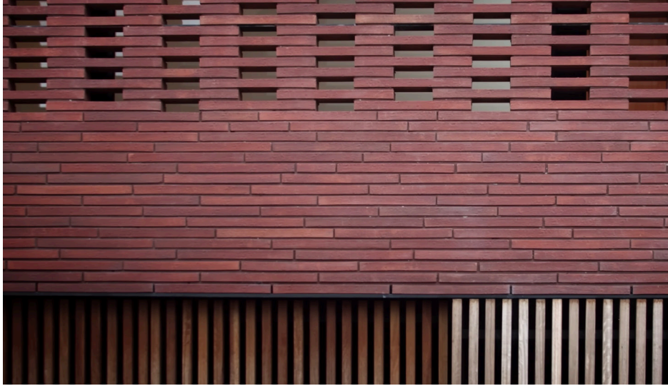
Figure 2.15 Northside House — Brick Exterior 2021
