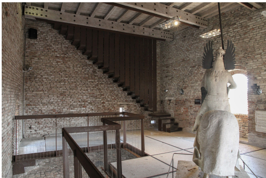
Figure 5.8 The Castelvecchio Museum's weathering steel staircase 1959-1973
