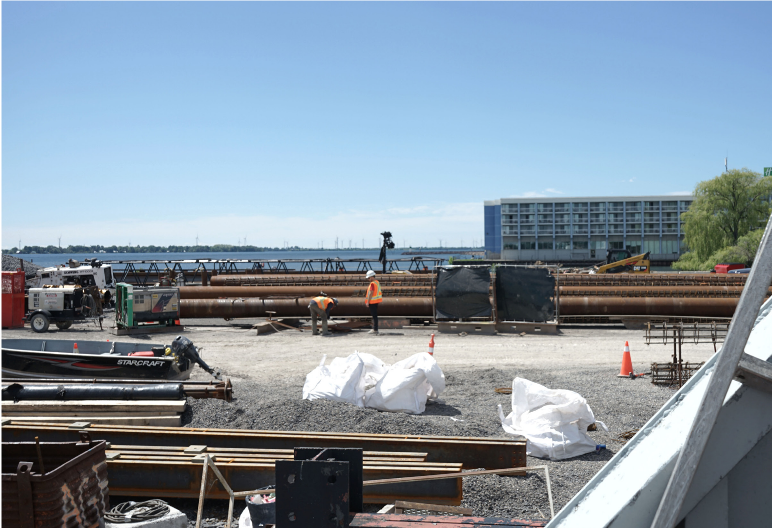
FIGURE 38 | CONSTRUCTION WOLFE ISLAND FERRY DOCK IN KINGSTON
