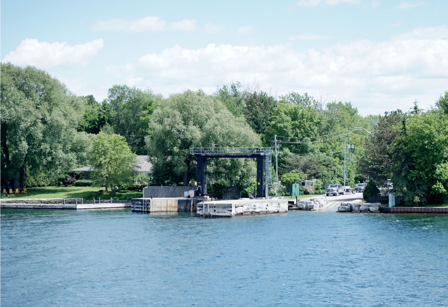
FIGURE 40 | HOWE ISLAND FERRY DOCK IN KINGSTON
