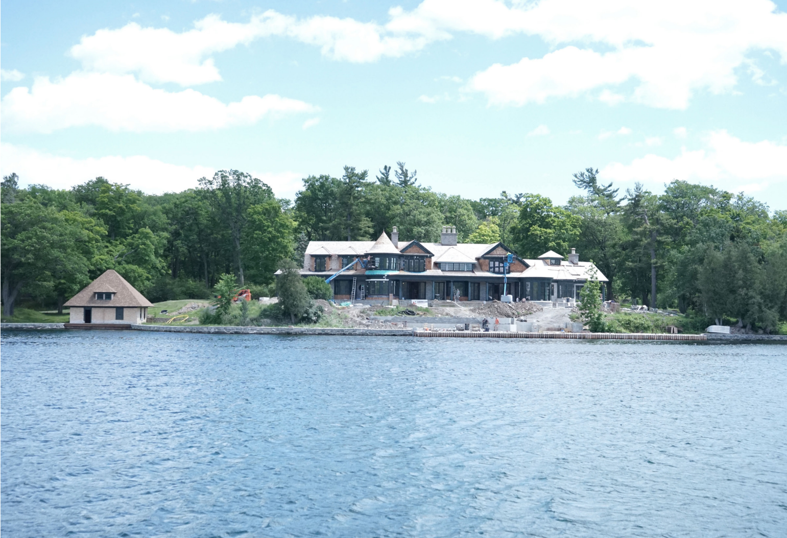
FIGURE 62 | WATERFRONT MANSION UNDER CONSTRUCTION
