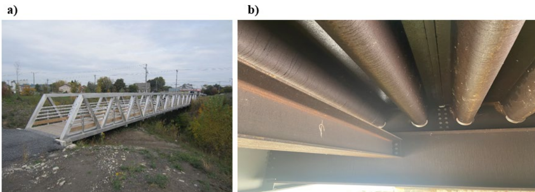
Figure 1.1: a) Aluminum pedestrian bridge in Brossard, QC, b) Murray Street Bridge OSD, ON.
