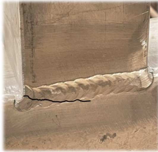
Figure 4.14: Actual weld crack propagation during an ongoing experiment starting from the edge of the specimen and propagating toward the opposite edge.
