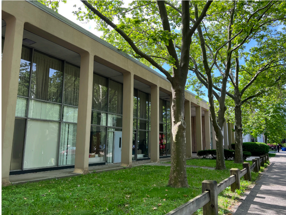
Fig. 4.4 Community centre, part of the Harry A. Conte Elementary School and Community Center, 15 Wooster Place.
