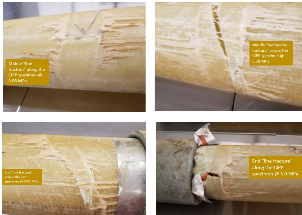
Figure 4.9: Examples of failure modes observed in the burst testing of the I-Main CIPP liner.
