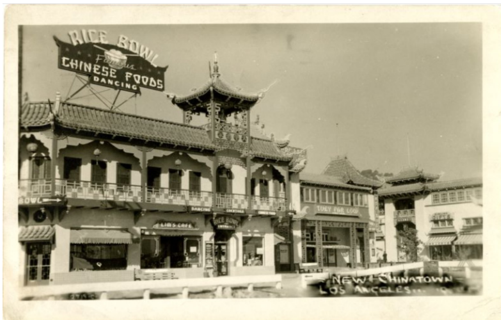
fig.2.24 View of Sun Mun Way on the west side of Central Plaza in New Chinatown, Los Angeles. (Werner von Boltenstern Postcard Collection)
