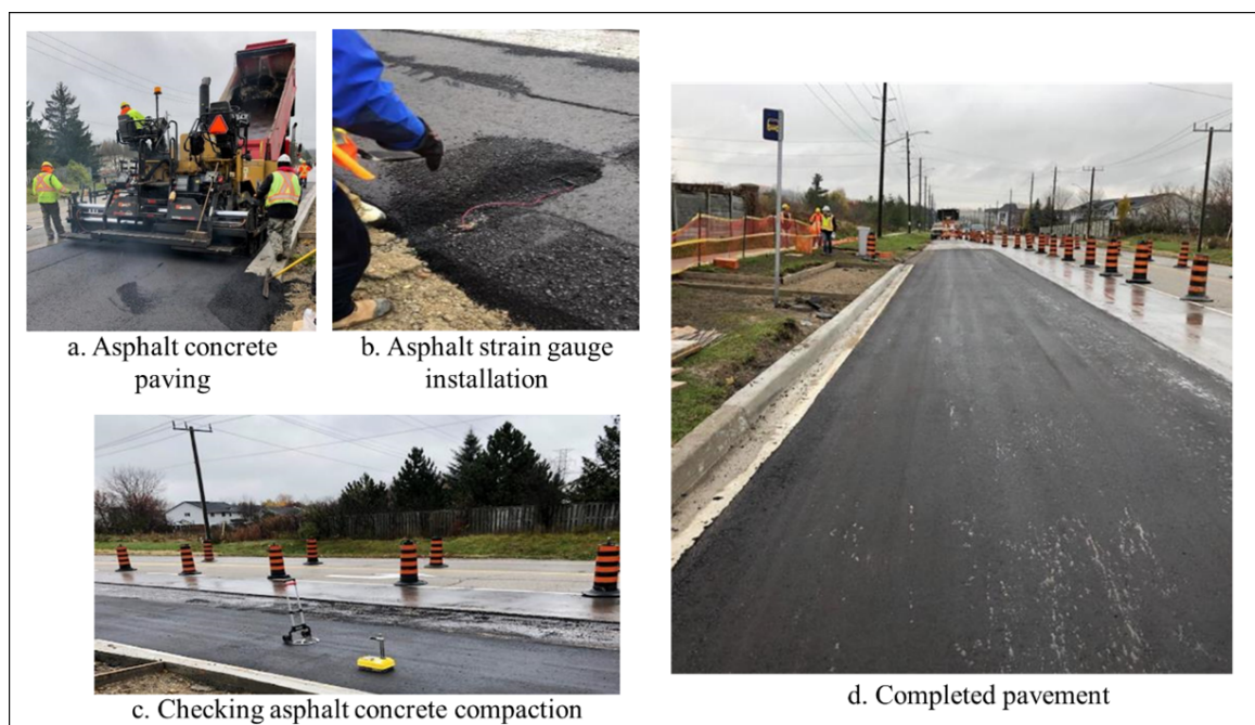
Figure 4.11: Asphalt concrete paving
