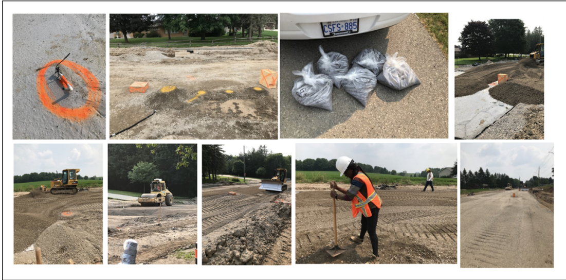
Figure 4.19: Sensor protection, granular A sampling, and placement
