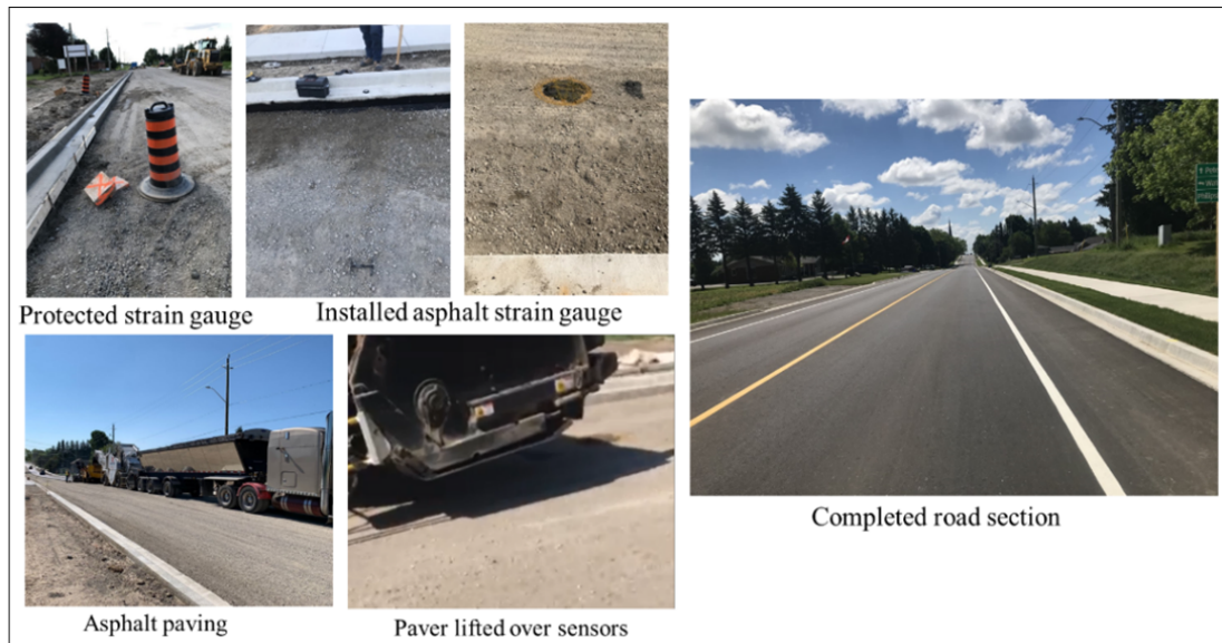
Figure 4.22: Notre Dame Drive asphalt concrete paving
