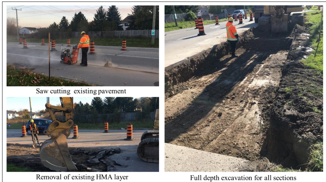
Figure 4.4: Site preparation and excavation
