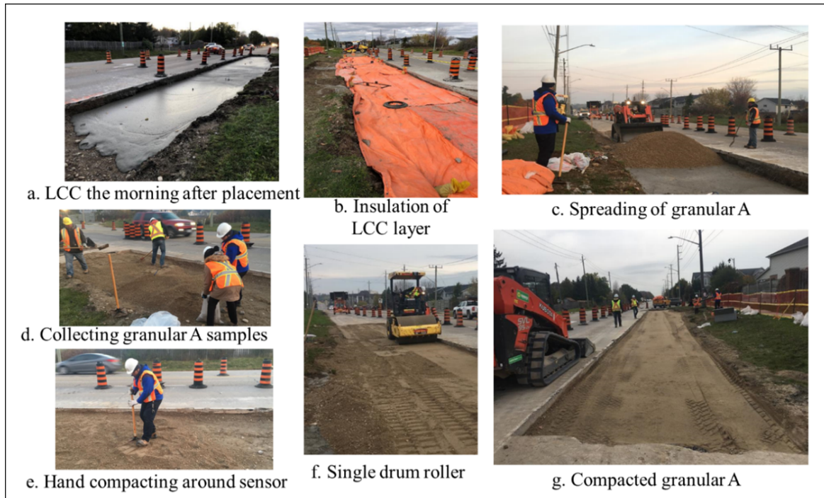
Figure 4.9: After LCC pour and base construction
