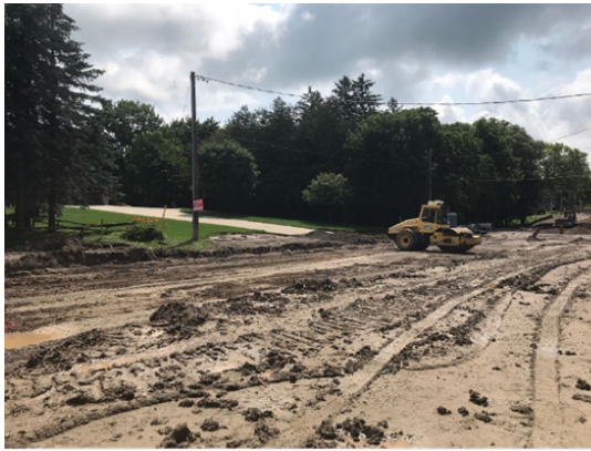
Overview of subgrade before construction
