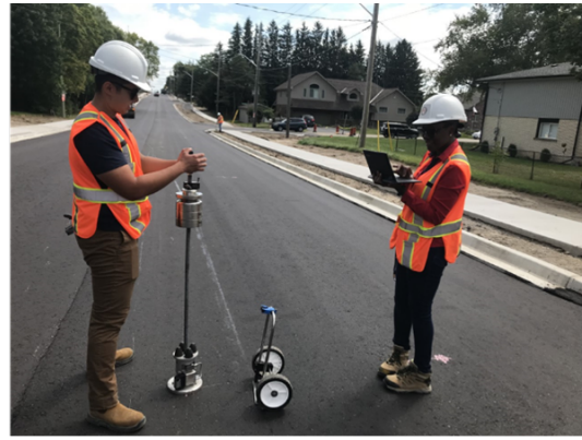
Lightweight Deflectometer testing at Notre Dame Drive
