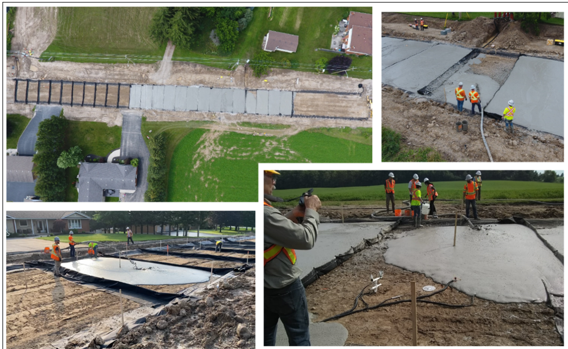
Figure 4.17: LCC pour and sampling
