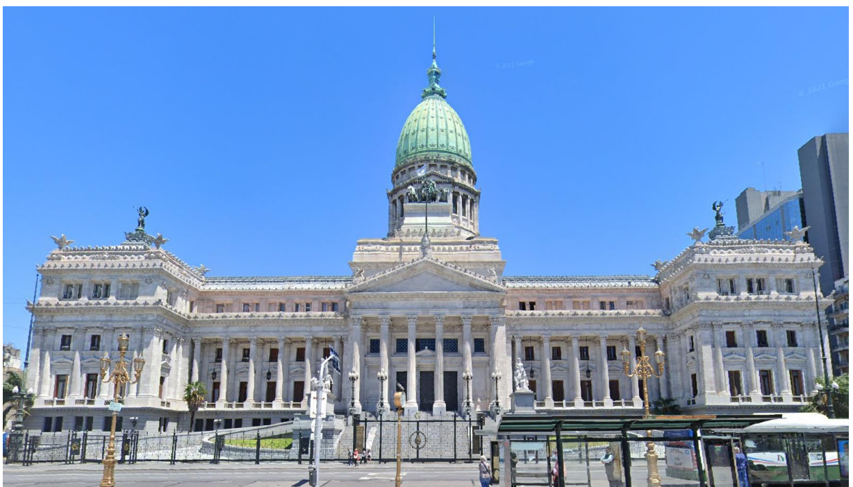
Built design with significant biomorphic (fractals; e.g., column details) and symmetrical ornamentation (Palacio del Congreso, Buenos Aires, Argentina, Photo from: Google Maps ©2021)
