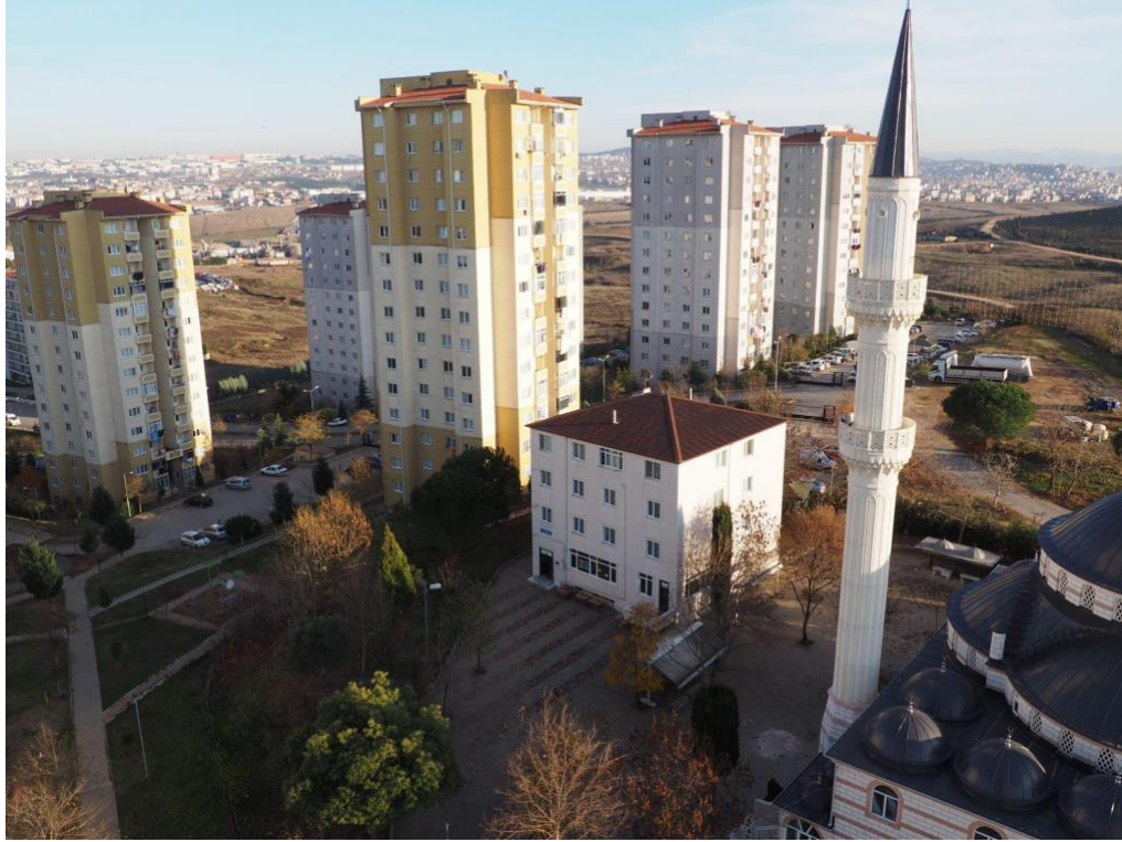
Figure 2.3. Aydınli TOKI Housing Estate and the mosque and the Quran course buildings Picture taken by the author, December 2019.
